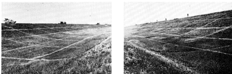
(a) View from top of backslope (b) View from ditch bottom
