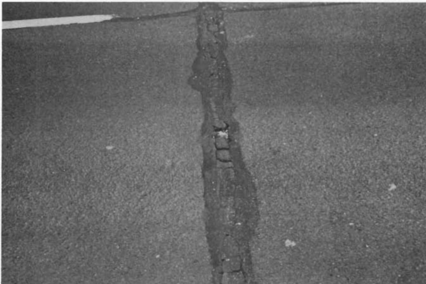
WITHOUT WIRE 200#/SY ACP OVERLAY
