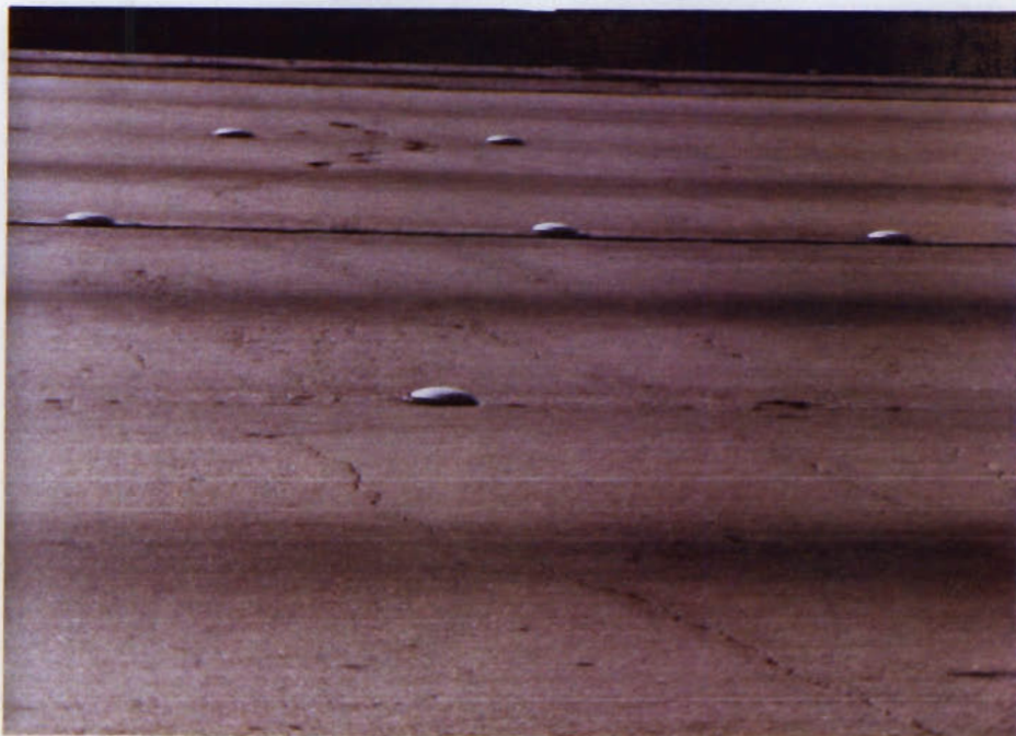
Figure 18: 1986 Contract Installation on I-45 (Gulf Freeway)
