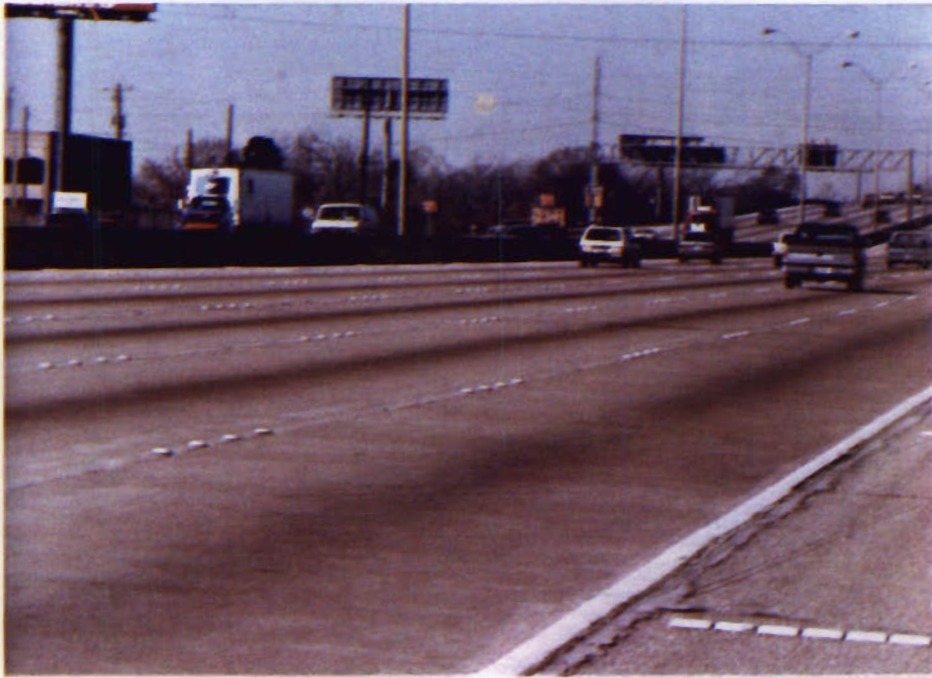
Figure 19: 1987 Contract Installation on I-10 (Katy Freeway)
