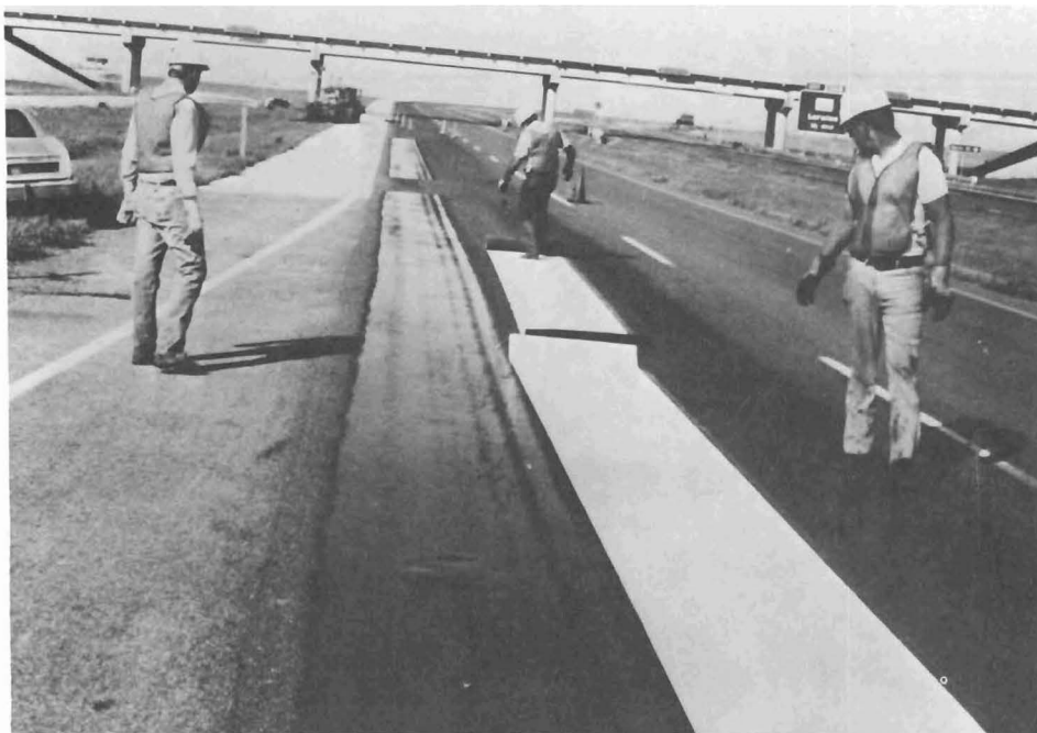
Placing and Walking down Rolled Roofing
