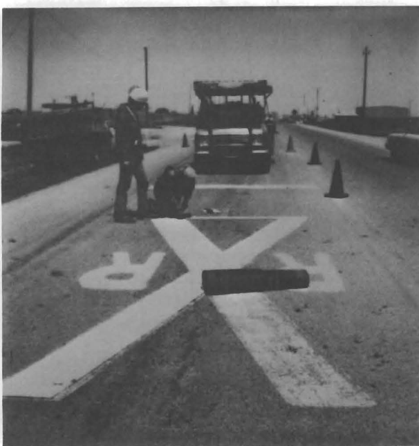
Completed Railroad-Highway Crossing Markings
