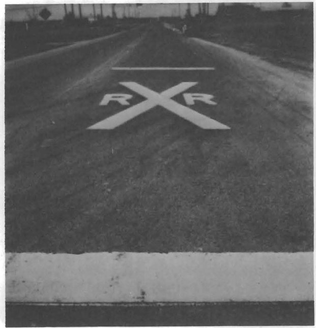
Completed Railroad-Highway Crossing Markings
