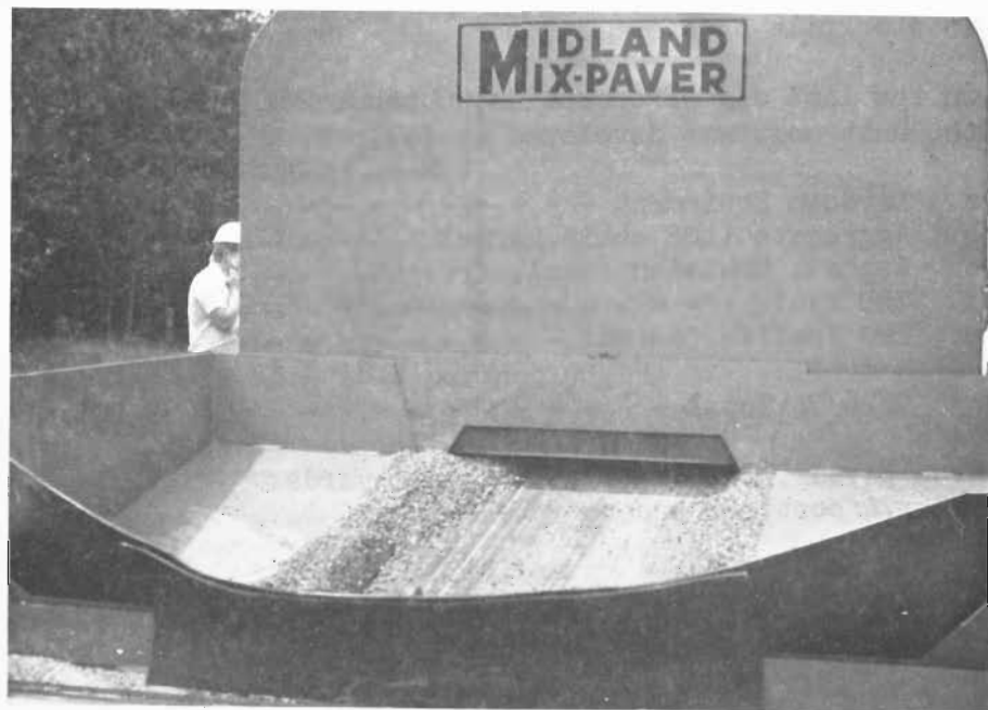
Figure 2 Hopper of Midland Mix-Paver showing adjustable entrance gate for uncoated aggregate
