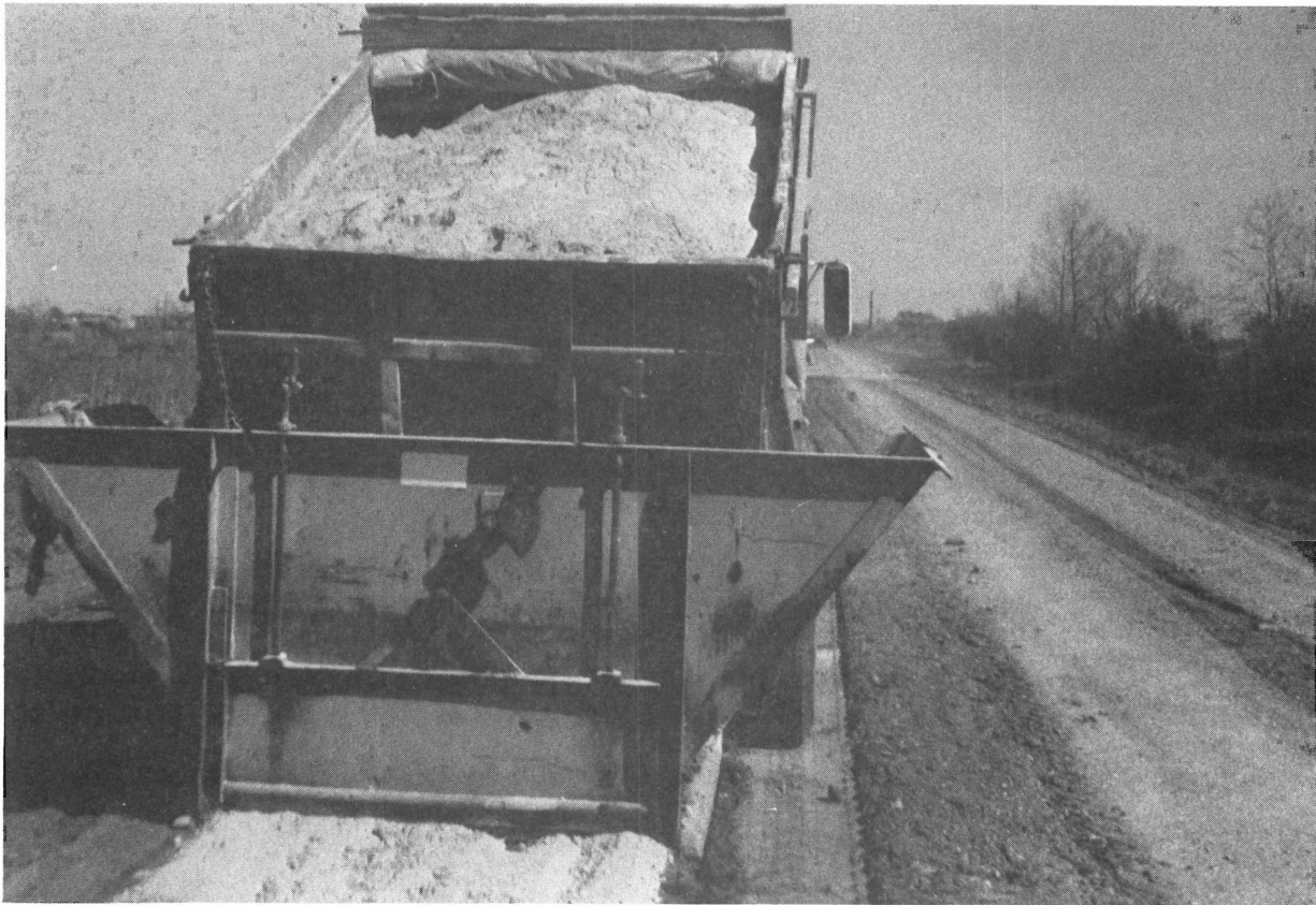
Figure 4: Stackdust being dumped through tailgate spreader
