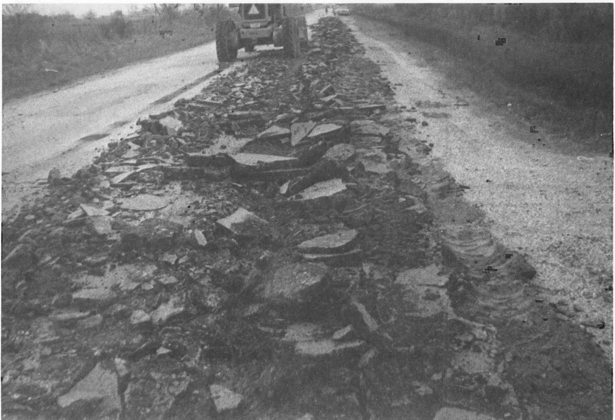
Figure 2: Scarifying old base and surface
