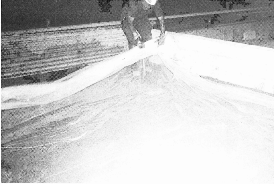
Figure 7. Placing Polyethylene Sheeting Over Monomer
