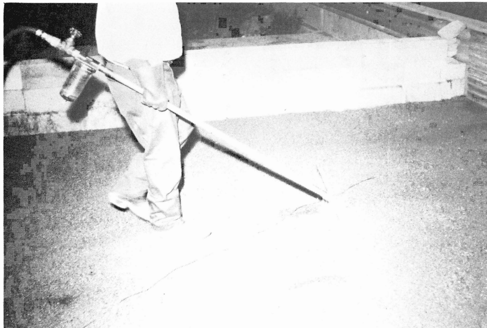
Figure 6. Placing Monomer
