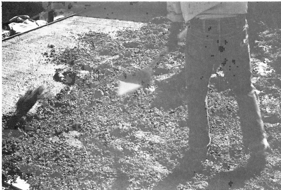
Figure 12. Spreading Overlay Concrete
