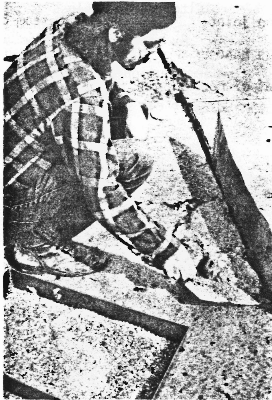
Figure 3 - Placing of Sand
