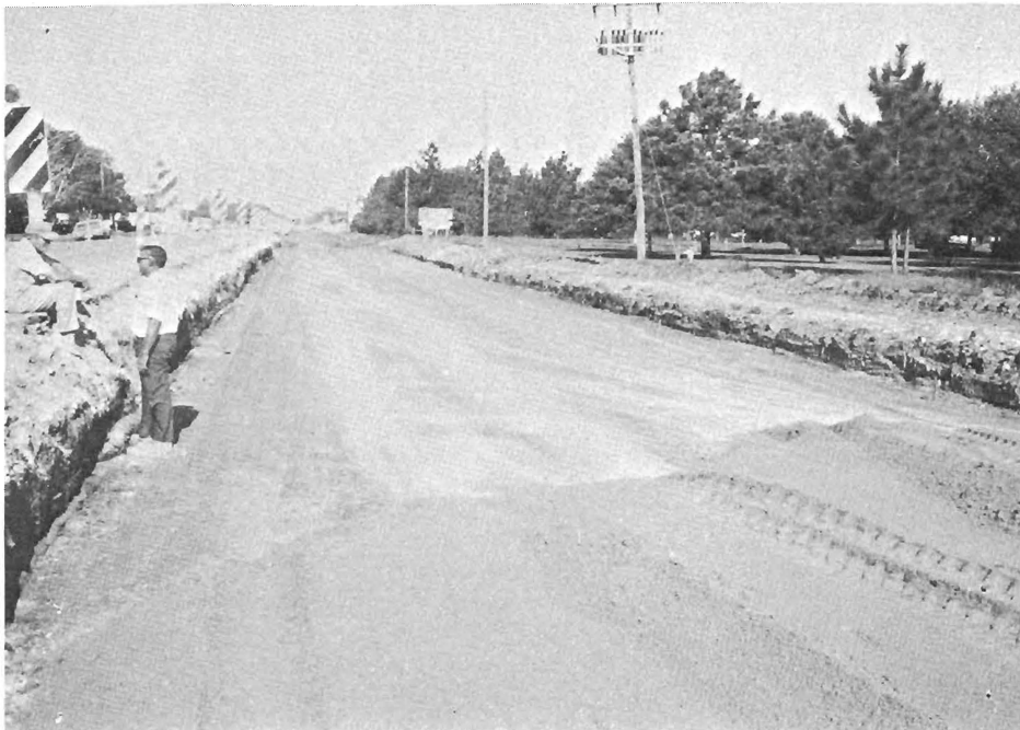
ChemComp expansive cement stabilized gravel screenings base on subgrade.
