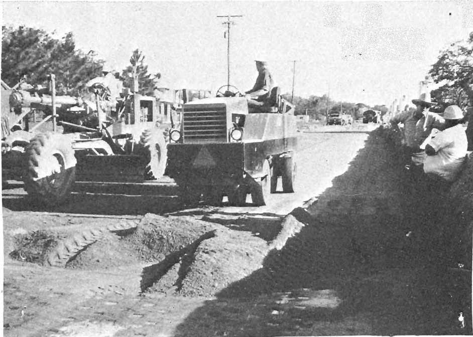
Grading and compacting cement stabilized base.
