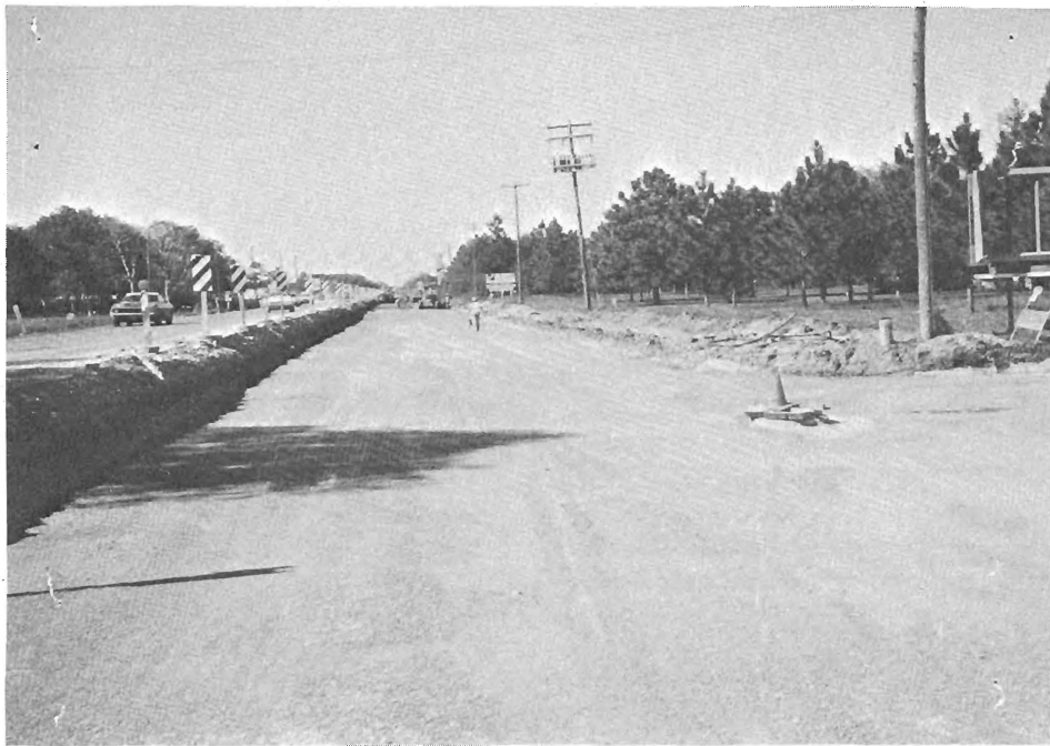
Curing 1st course of cement stabilized base
