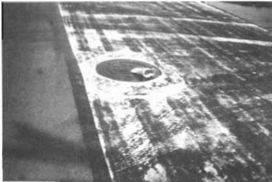
CLOSE-UP FABRIC UNDERSEAL PLACEMENT AT TYPICAL MANHOLE LOCATION.
