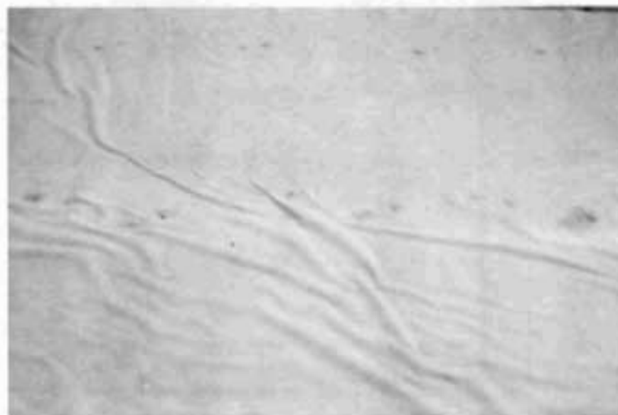
FABRIC UNDERSEAL IMMEDIATELY AFTER PLACEMENT SHOWING TYPICAL WRINKLING.
