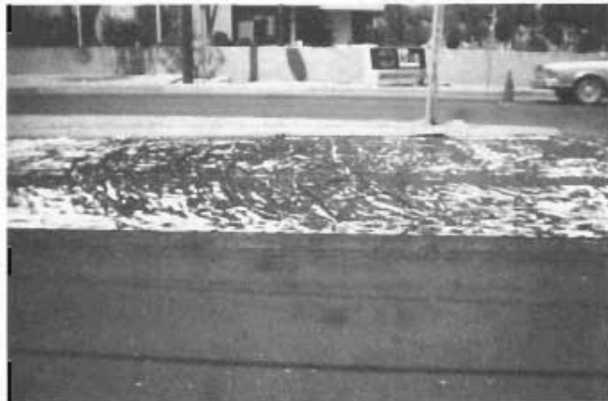
APPEARANCE OF FABRIC UNDERSEAL WITH NOTICEABLY MORE ABSORPTION OF AC-10 AND WRINKLING THAN IN MOST OTHER PLACES.
