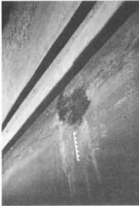
- TEST CORE NO. 3- AT SLIPPAGE AREA NO. 2
