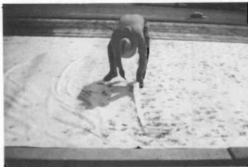
THE MORE SEVERE WRINKLES WERE CUT OUT WITH A POCKET KNIFE ALLOWING FABRIC TO LAY FLAT.
