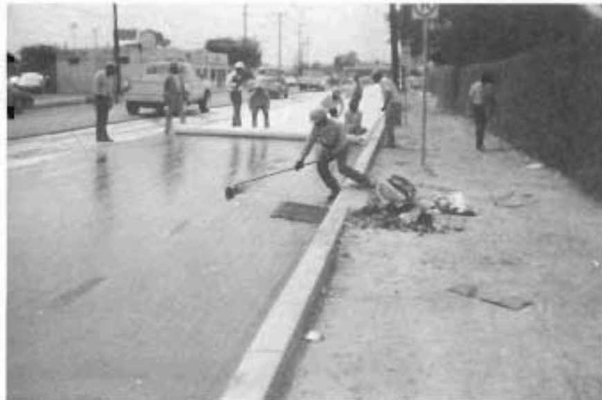
FABRIC UNDERSEAL BEING PLACED ON FRESHLY LAID AC-10 ASPHALTIC MATERIAL.
