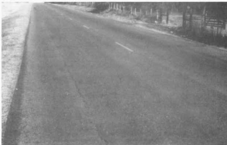
FIGURE 14 - VIEW OF SECTIONS 3 AND 4 IN FIRST WINTER - 7 MONTHS 10
