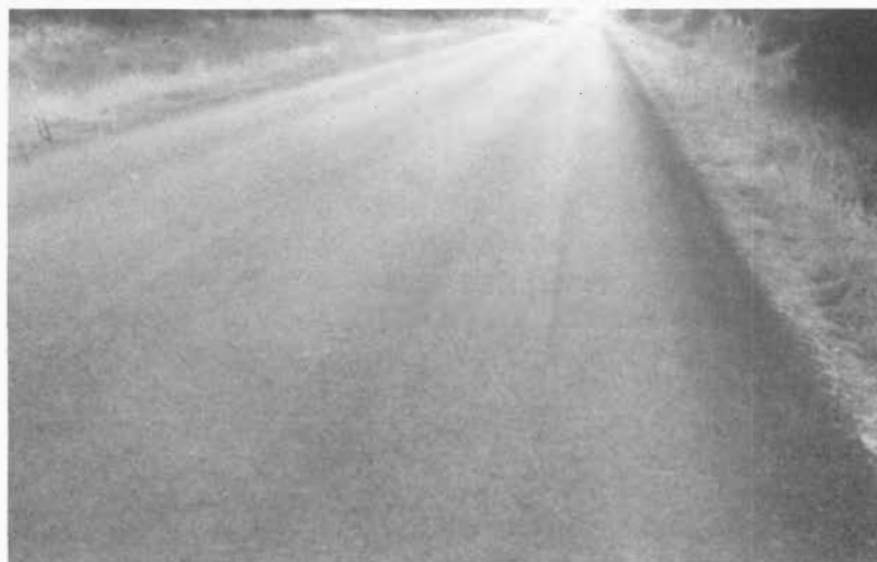
FIGURE 7 - GENERAL VIEW OF SECTIONS 3 AND 4
