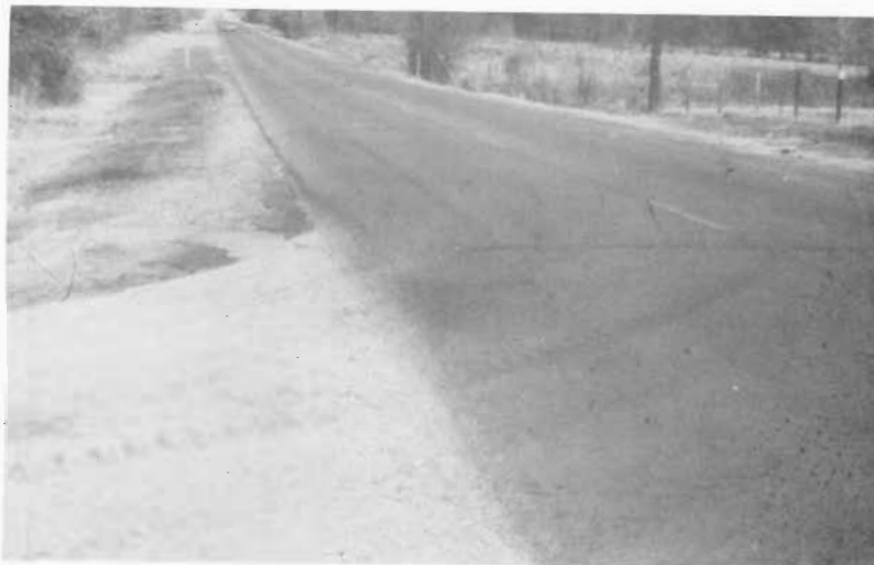
FIGURE 17 - VIEW OF SECTIONS 5 AND 6 IN FIRST WINTER - 7 MONTHS
