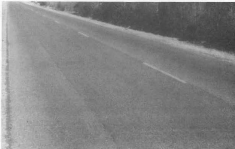
FIGURE 11 - VIEW OF SECTIONS 1 AND 2 IN FIRST WINTER - 7 MONTHS
