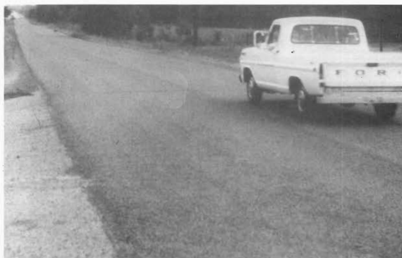
FIGURE 8 - GENERAL VIEW OF SECTIONS 5 AND 6
