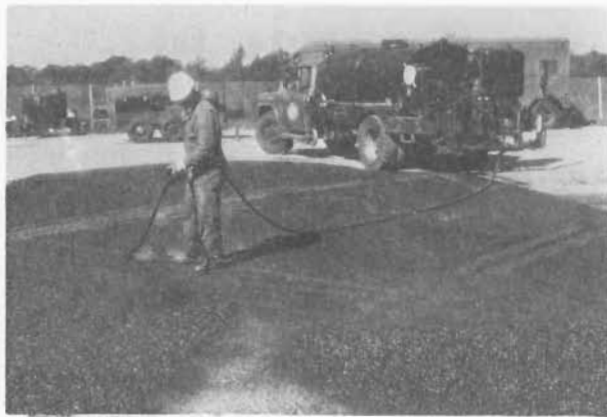
"Sweetening Precoated Material With Emulsion In Maintenance Yard
