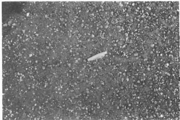
Completed Section Of Sprinkle Treatment
