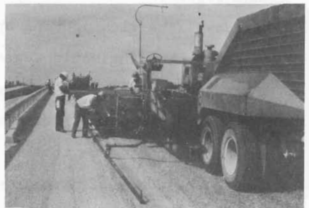
Laydown Machine In Foreground Aggregate Spreader In Background
