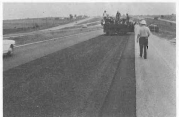
Aggregate Spreader Applying Sprinkle Treatment
