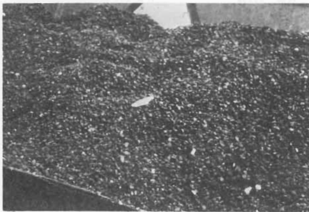
Asphalt Coated Aggregate In Hopper Of Spreader Ready For Sprinkling
