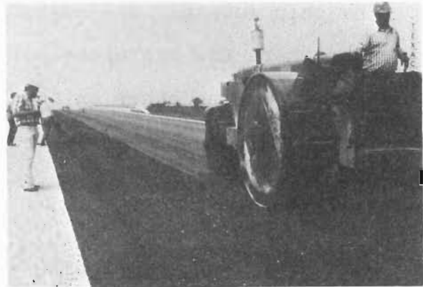
Rolling With Three Wheeled Roller In Progress
