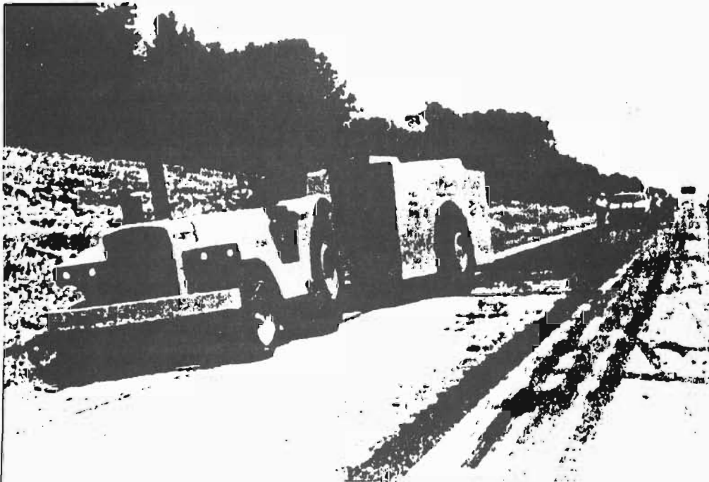
A 27,216 to 45,359 kg (30 to 50 Ton) Proof Roller Is Used for Seating.
