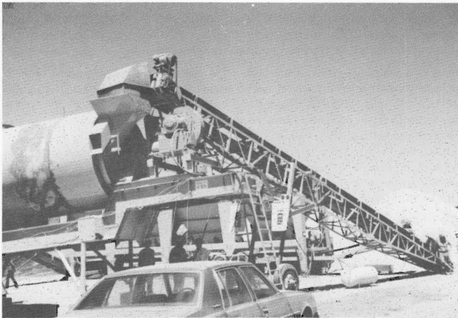
Figure 4.14. Inclined conveyor.
