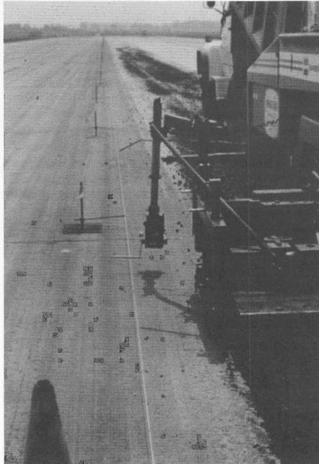
Figure 13.4. Erected stringline.
