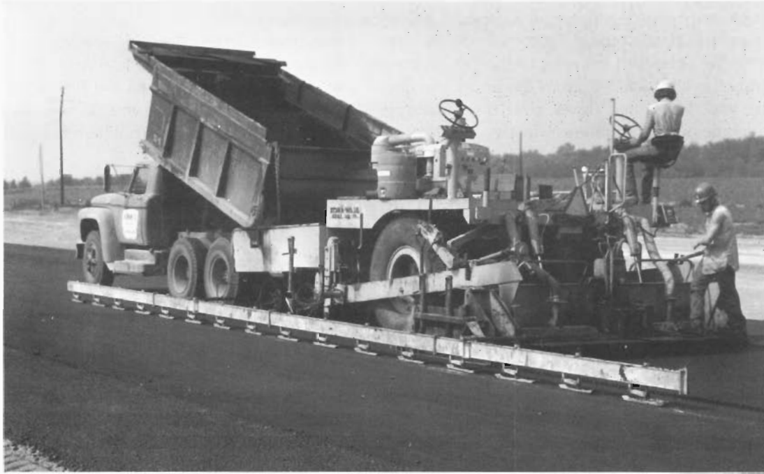
Figure 13.6. Floating beam grade reference.
