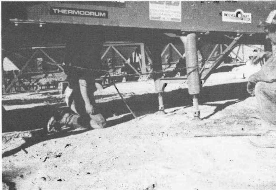
Figure 7.18. Changing slope of the drum.
