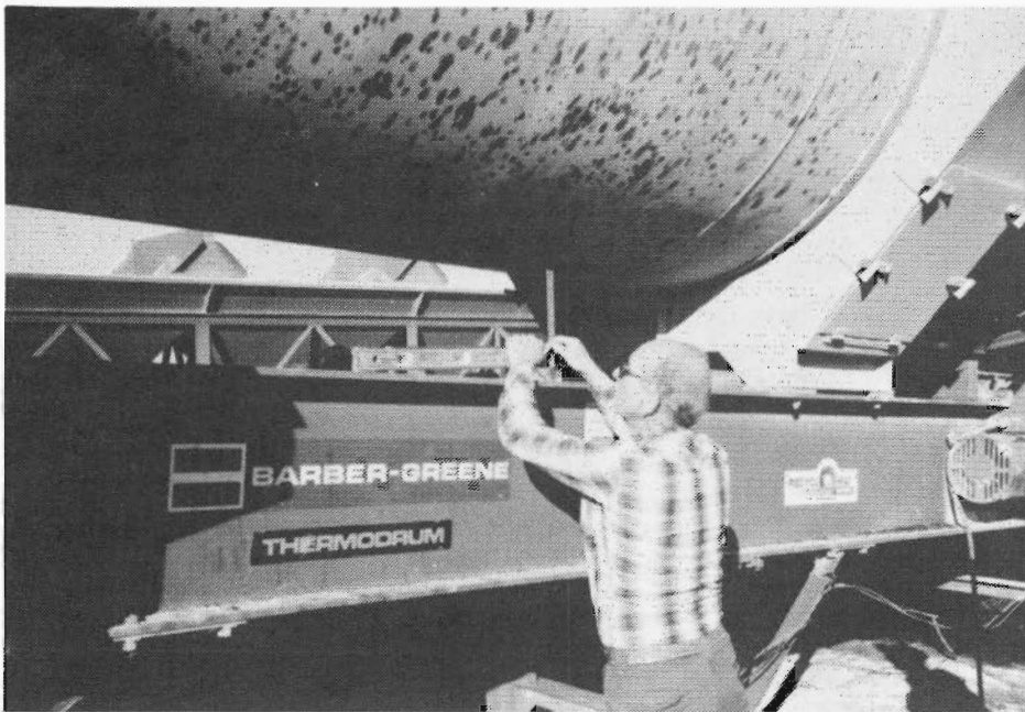
Figure 7.19. Changing slope of the drum.
