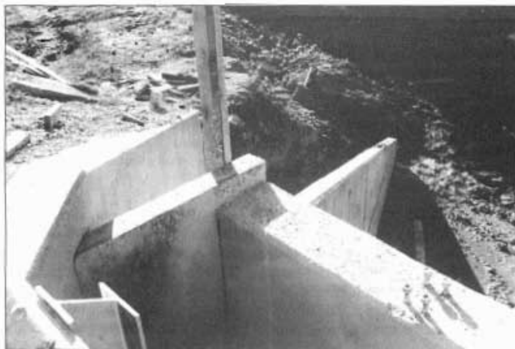
FIGURE 7: Forms at Side of New Headwalls
