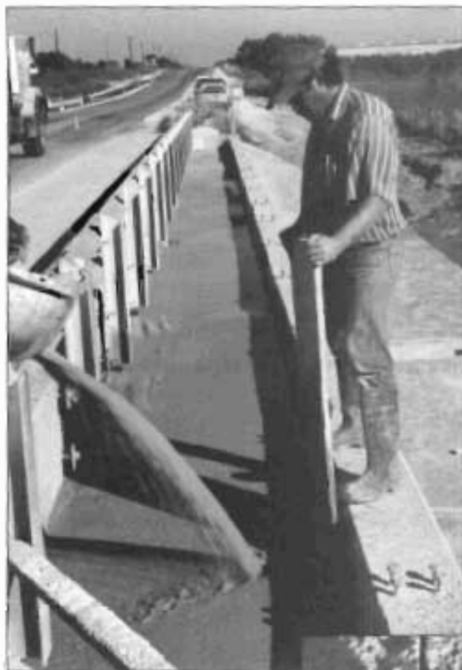
FIGURE 5: Flowable Fill Placement
