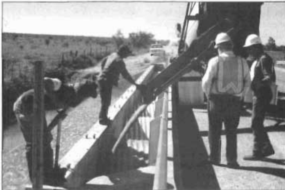
FIGURE 4: Flowable Fill Placement
