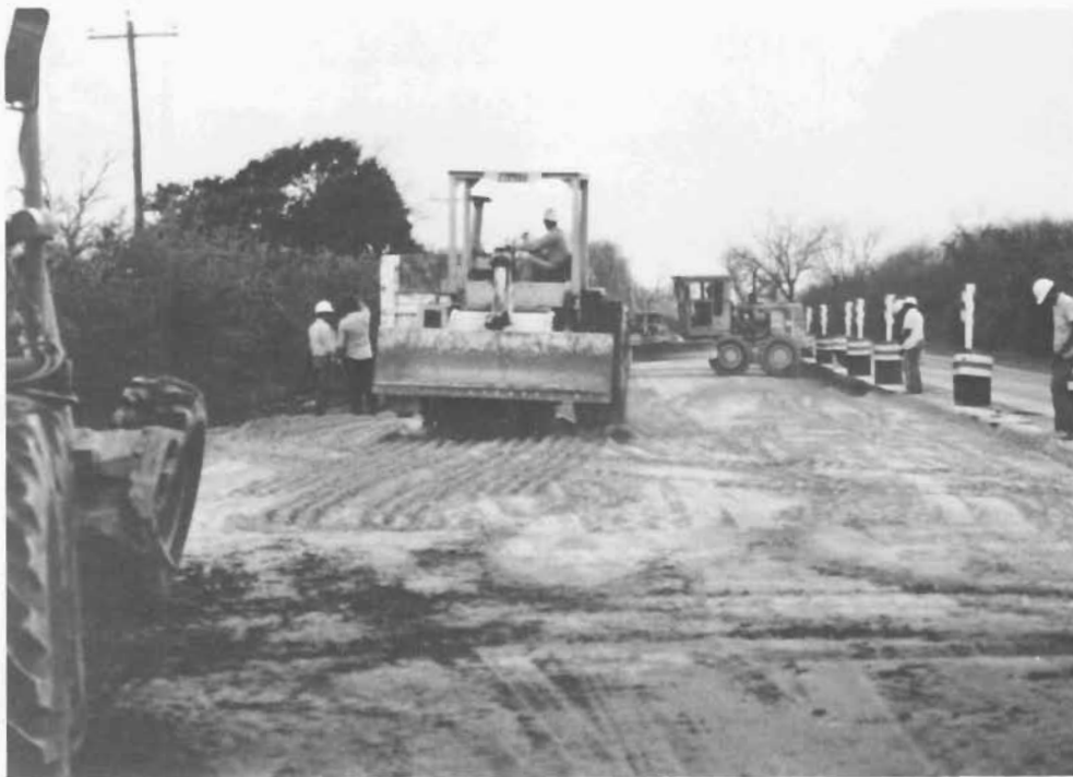
In this picture, taken on March 29, 1988, fly ash is being compacted.
