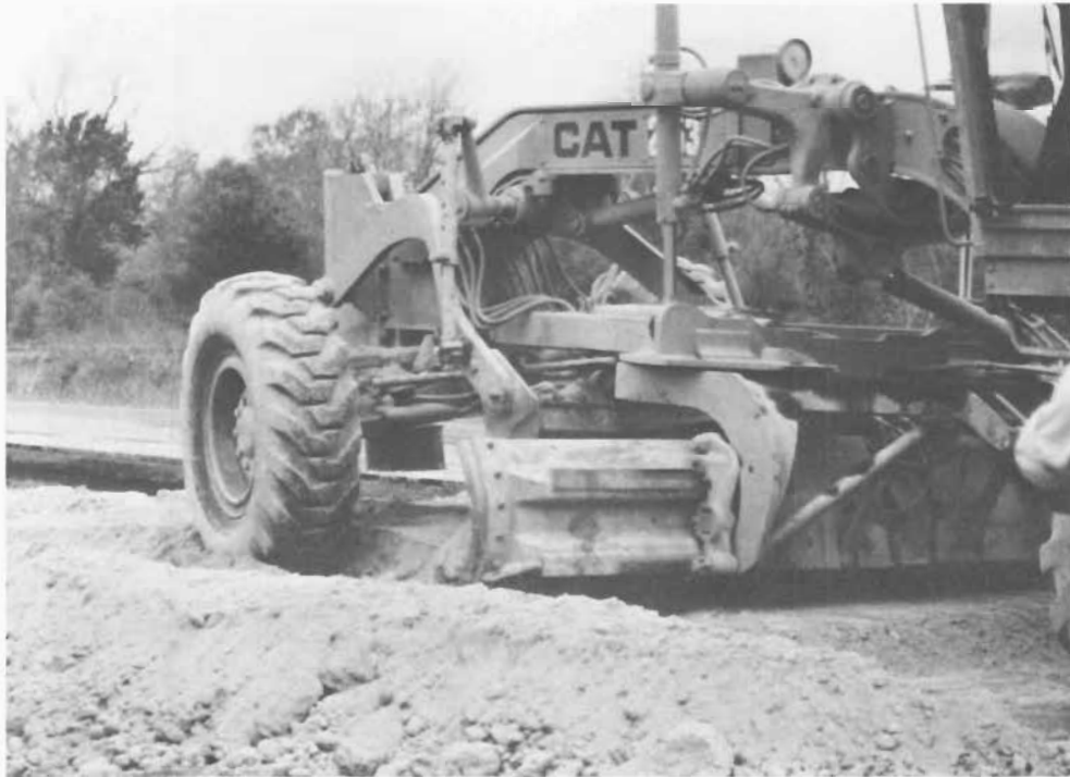
Fly ash is being leveled off in this picture taken on March 29, 1988.
