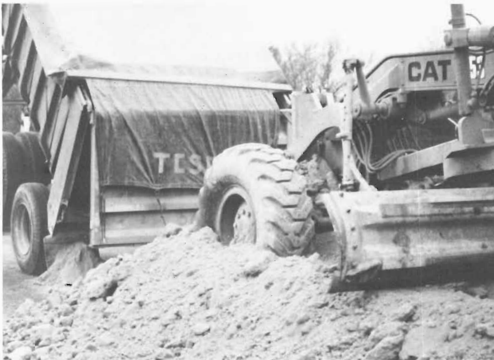
This picture shows fly ash that was just dumped being leveled off on March 29, 1988.
