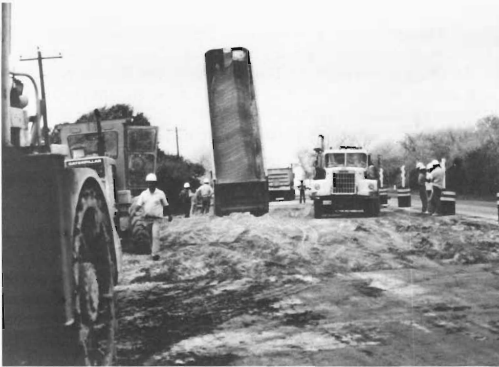
This picture, taken March 29, 1988, shows that it was difficult to get the fly ash out of the dump truck. Here the hydraulic lift on the truck was up all the way, yet the fly ash was still in the truck.
