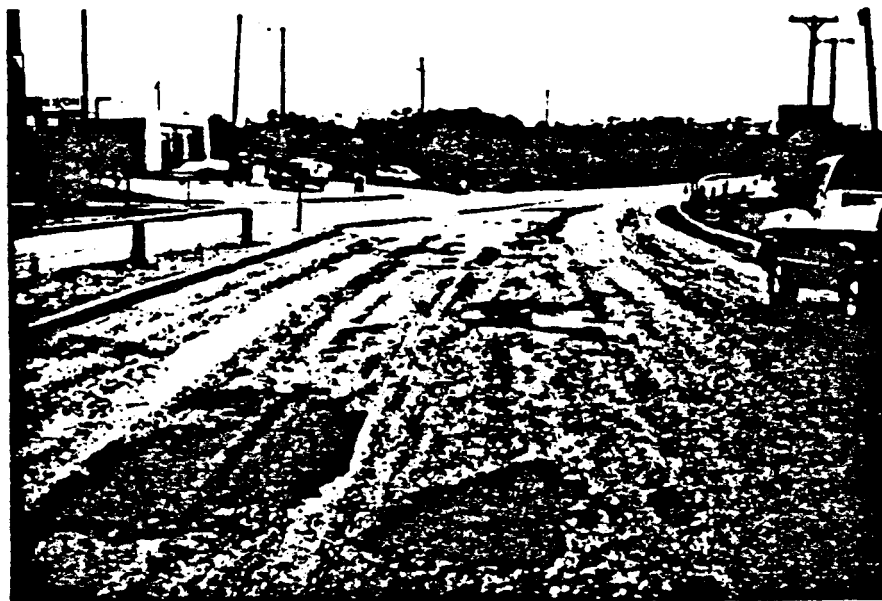
SHOVED AREAS AFTER REPAIRS
