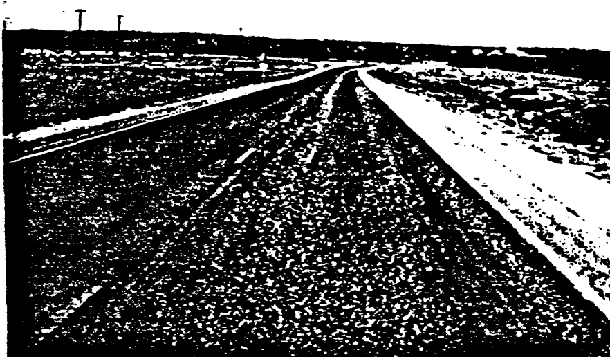
PRONOUNCED STREAKING IN UNOFFICIAL (1980) SULPHLEX SEAL COAT
