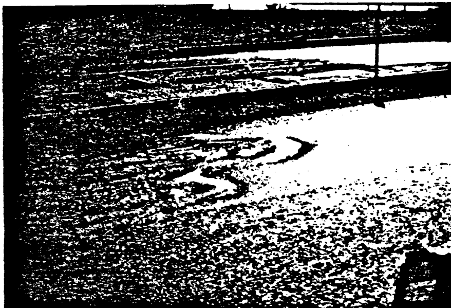
SHOVED AREAS BEFORE REPAIRS
