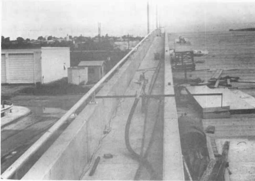
PEDESTRIAN SIDEWALK AND NATURAL GAS AND WATER LINES
