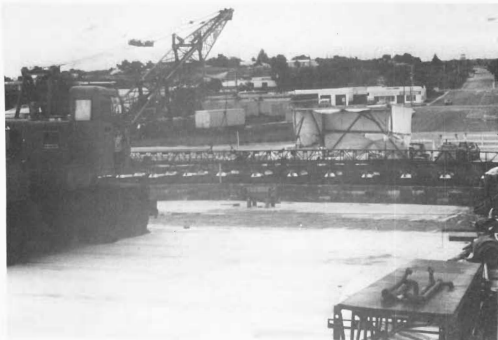
HEATERS IN POSITION FOR DRYING
