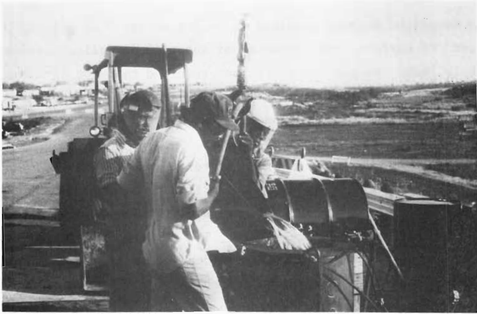
MIXING THE MONOMER SYSTEM
