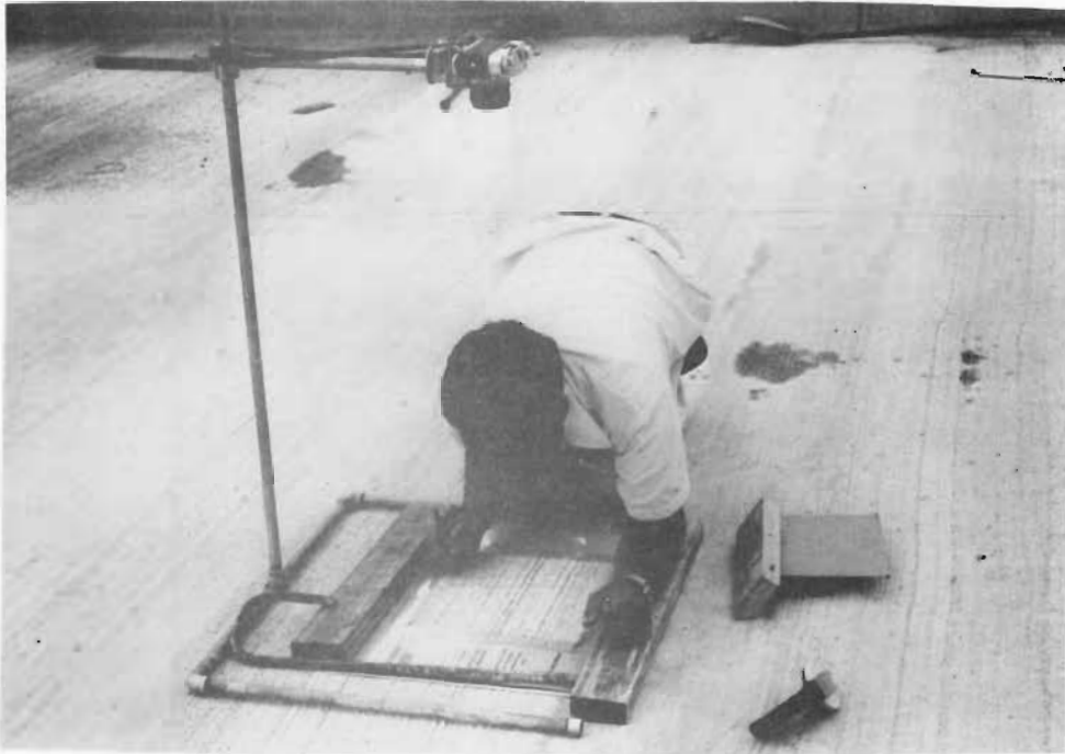
MAKING CRACK SURVEY AND PHOTOGRAPH
