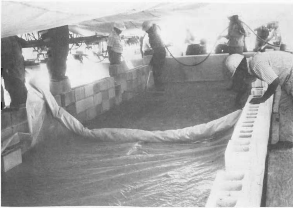
PLACING MONOMER AND COVERING POLYETHYLENE SHEETING
