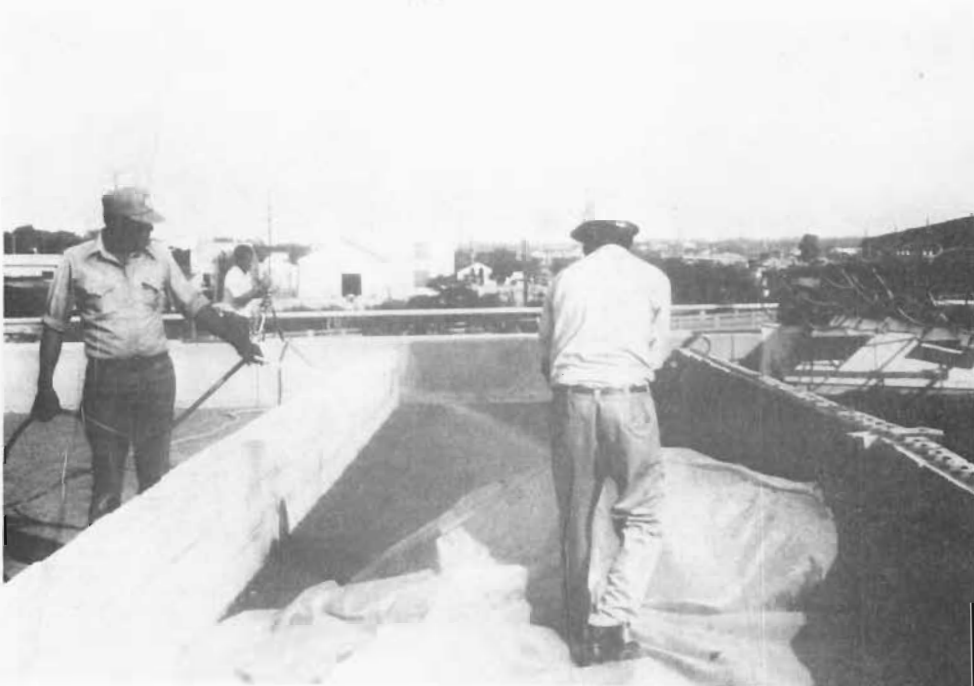
REMOVING POLYETHYLENE SHEETING AND SPRINKLING WITH WATER AFTER SOAKING
