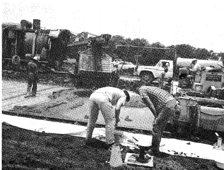
FIGURE 2.12 Placing Concrete
