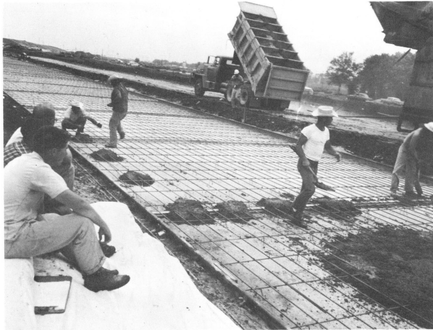
FIGURE 2.13 Covering Instrumentation with Concrete Ahead of General Operations
