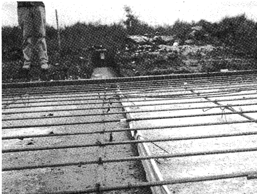
FIGURE 2.6 Strain Gage Installation
