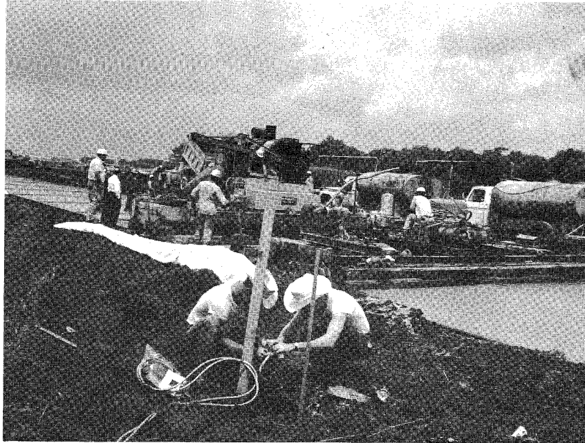
FIGURE 2.11 Paving Operations in Progress
