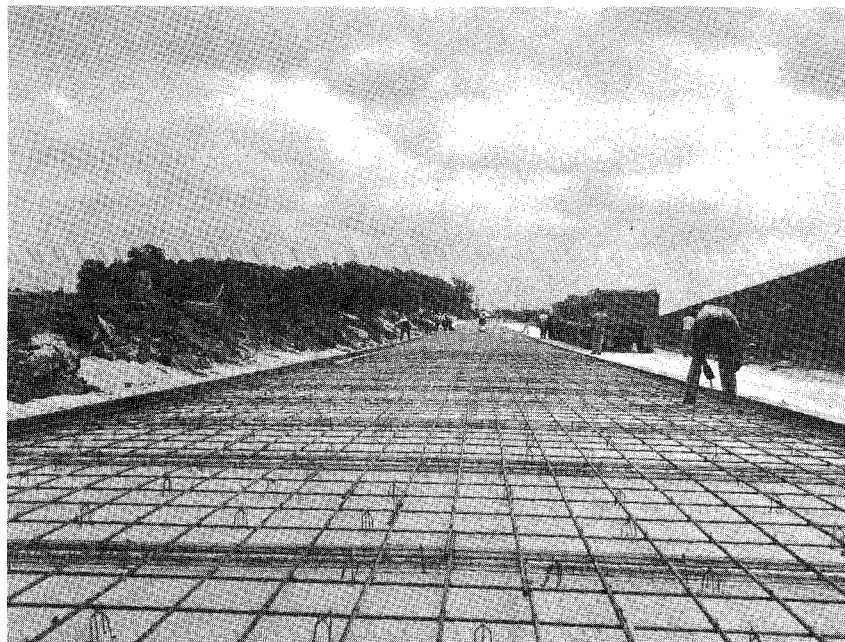
FIGURE 2.8 Construction for Preformed Cracks
