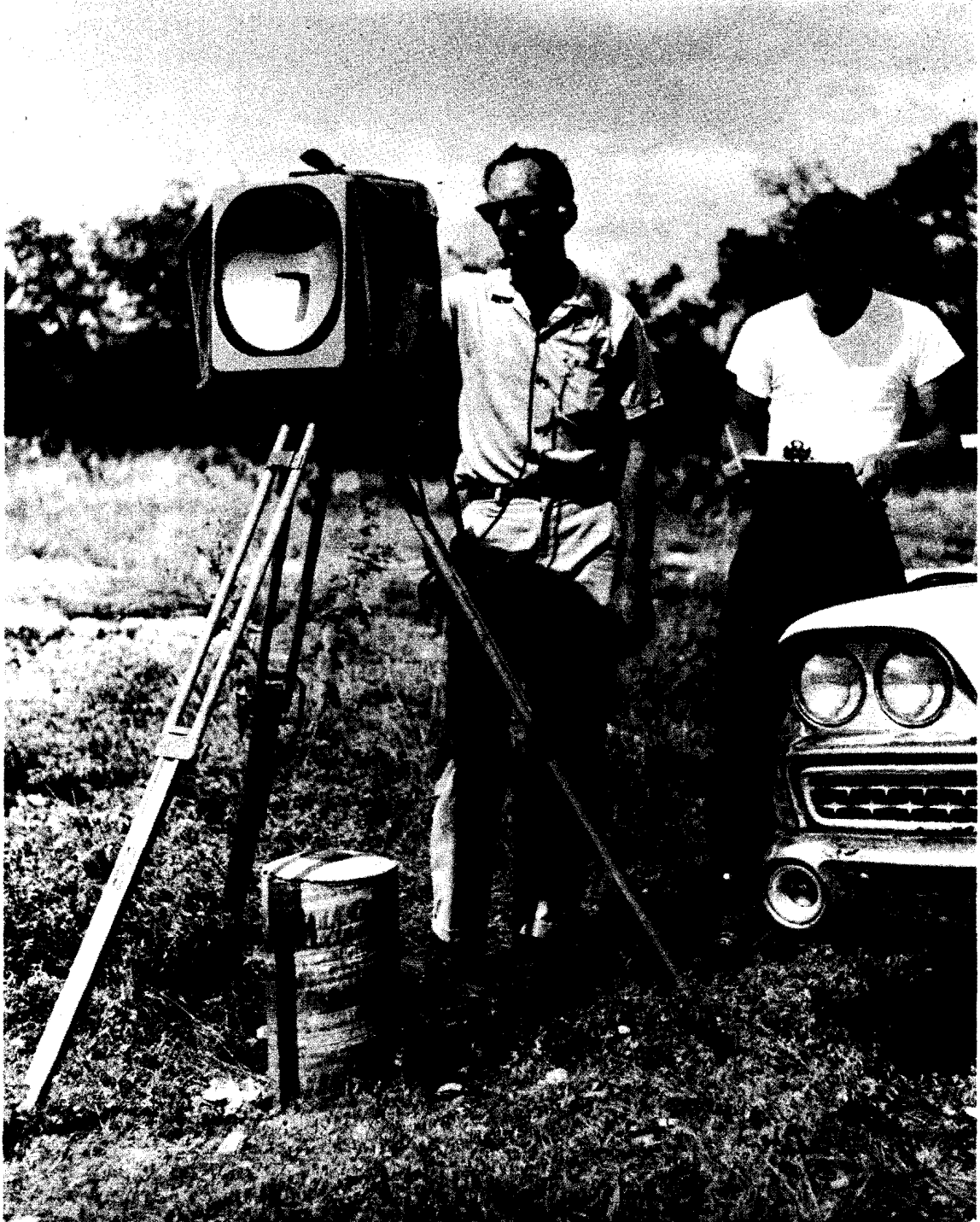
Figure 3. Electrotape Measuring On The Mile Baseline
