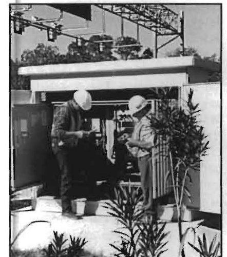
FIG. 5: Working on a fiber hub cabinet. (Credit: Kemp Davis Photography)
