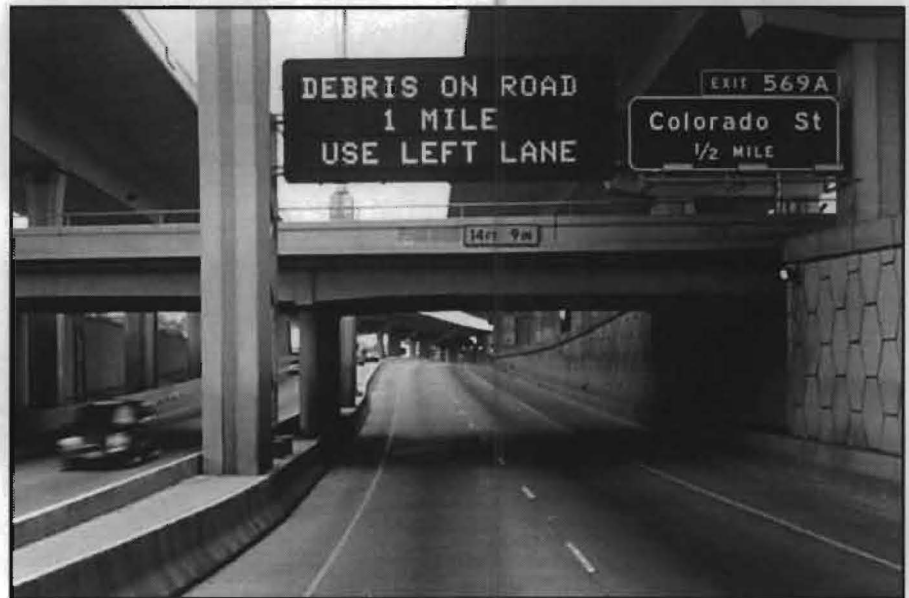
FIG. 1: A variable message sign, part of the TransGuide System, warns motorists of changing freeway conditions. (Credit: Kemp Davis Photography)
