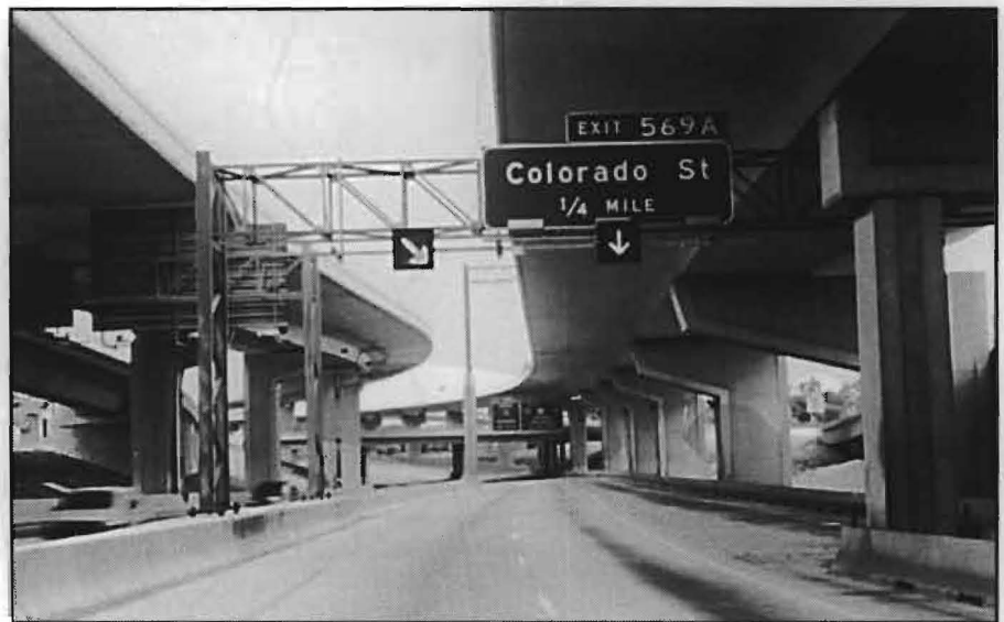
FIG. 7: Lane control signals. The left-hand one is a diagonal yellow, warning motorist to merge with the right lane. The down arrow in the right-hand lane is green, showing the lane is open and traffic is running normally. (Credit: Kemp Davis Photography)
