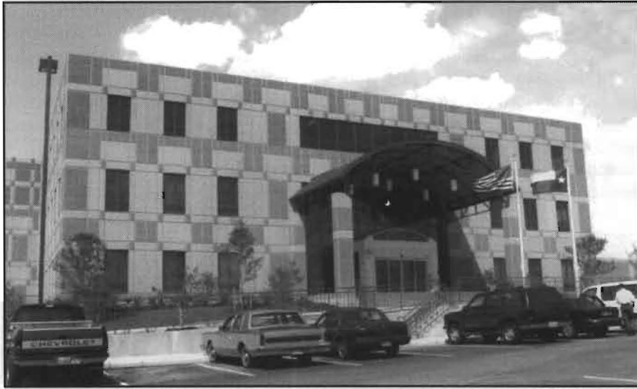
FIG. 2: San Antonio District's TransGuide operations center. (Credit: Bill Frost, SAT, TxDOT)
