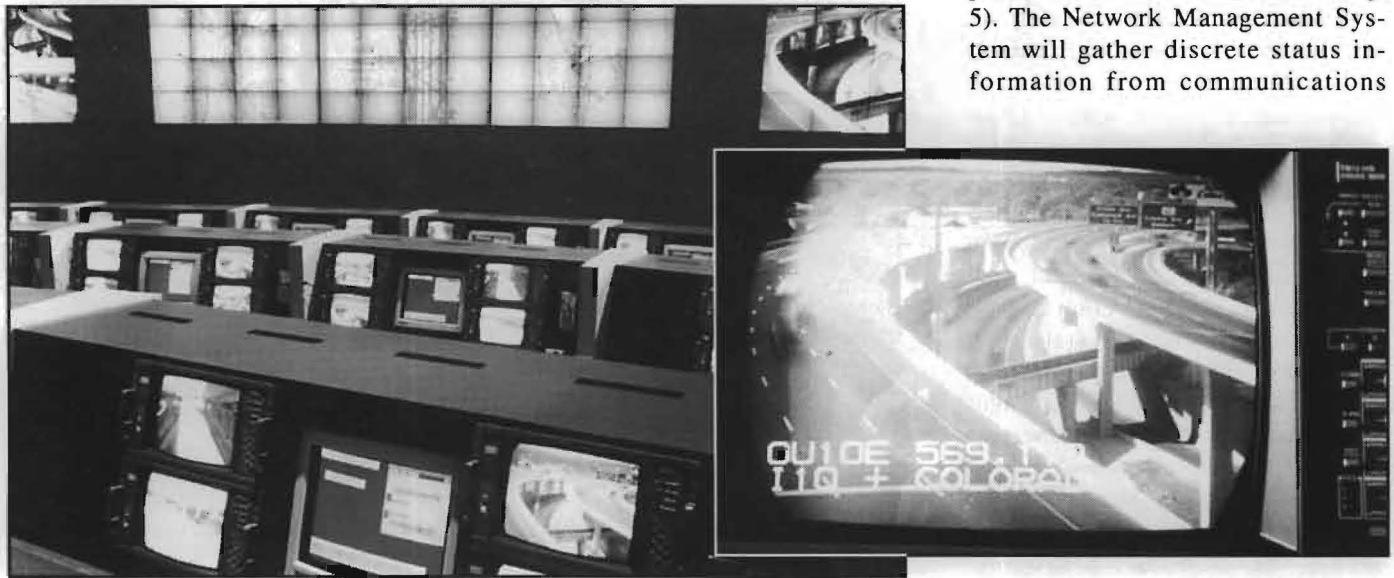
FIG. 3: View of the video wall in the operations room. Inset shows close-up of workstation screen. (Credit: Kemp Davis Photography)
