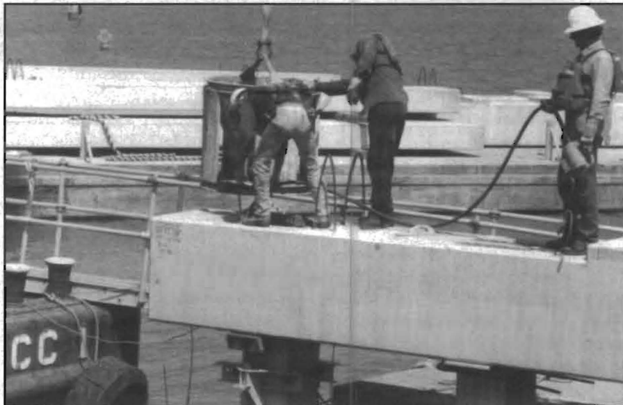
FIG. 4 : Filling slotted voids with concrete and vibrating into place.
