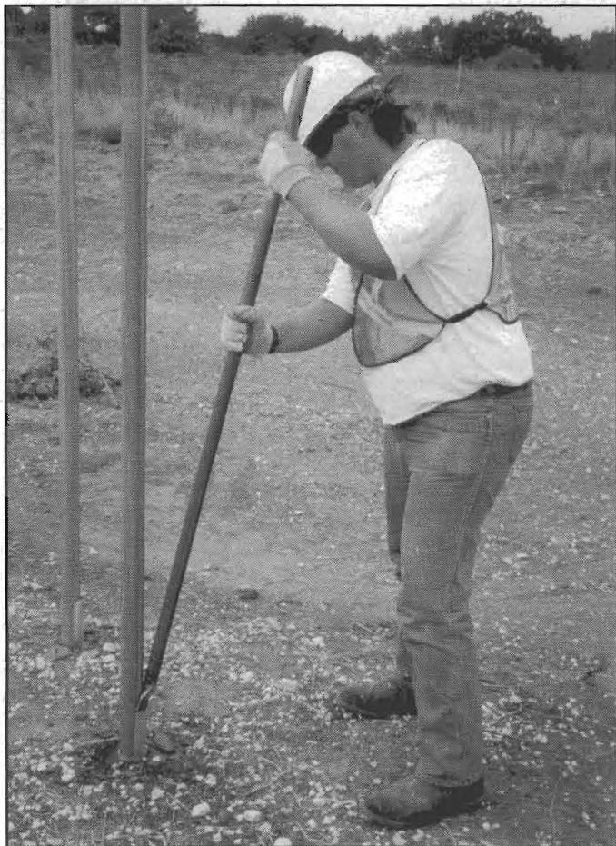
FIG. 2: The bar allows a worker to stand while driving in the POZ-LOK wedge.
