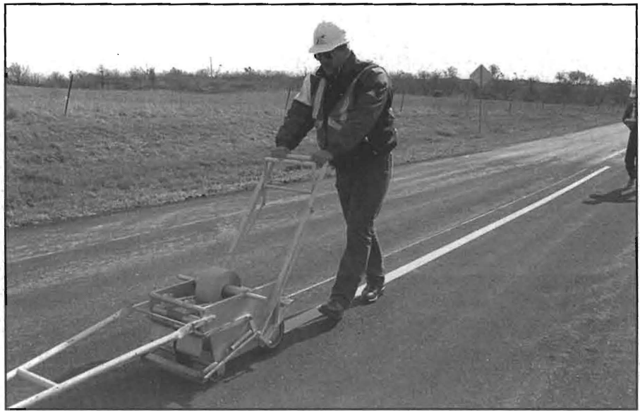
FIG. 1: Applying permanent tape stripe to a fresh premix patch on FM 619.
