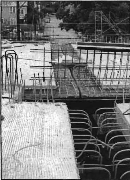
FIG. 13: Slab C9 poor-boy closure.
