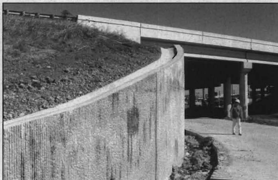
FIGURE 1: The completed soil nail wall on IH 30 at SH 205.
