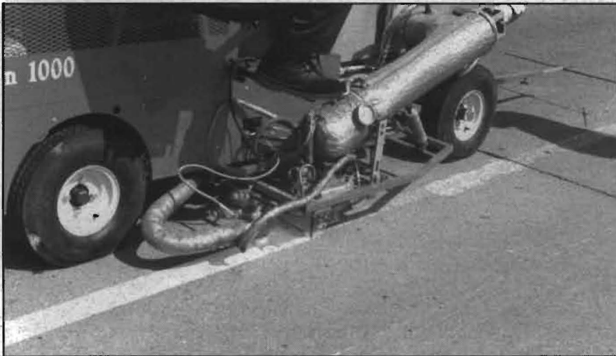
FIGURE 2: Forming the ridges within the stripe with a modified extruder.
