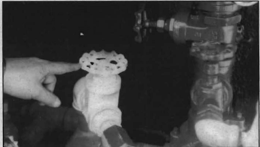
FIGURE 4: Suction valve (white) — valve in open position transfers material from flush tank to reservoir or back to distributor.
