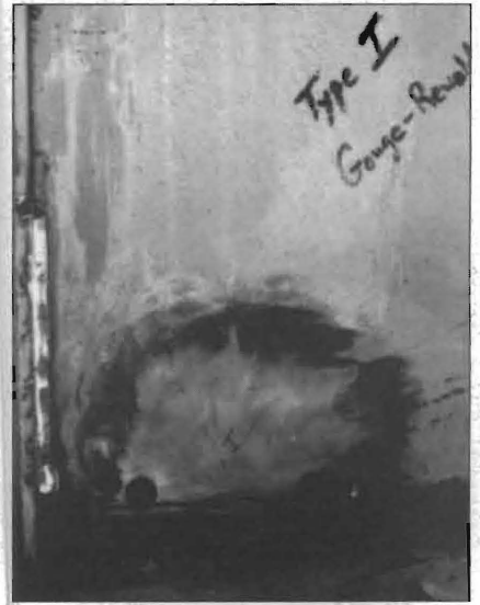
FIG. 12: Typical finished type 1 repair.
