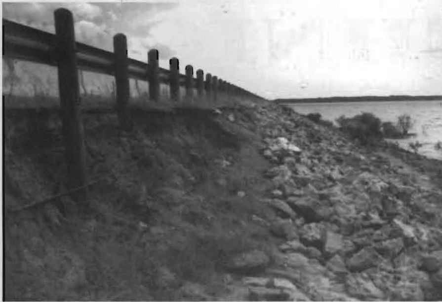
FIGURE 2A: SH 147 embankment, Sam Rayburn Reservoir, District 11.
