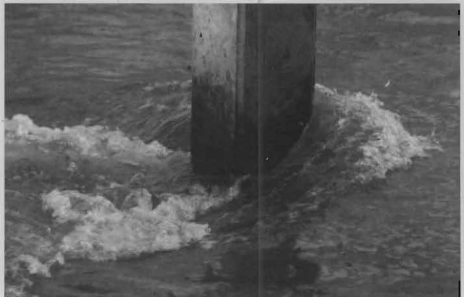
FIGURE 1: Turbulence may indicate scour at columns.
