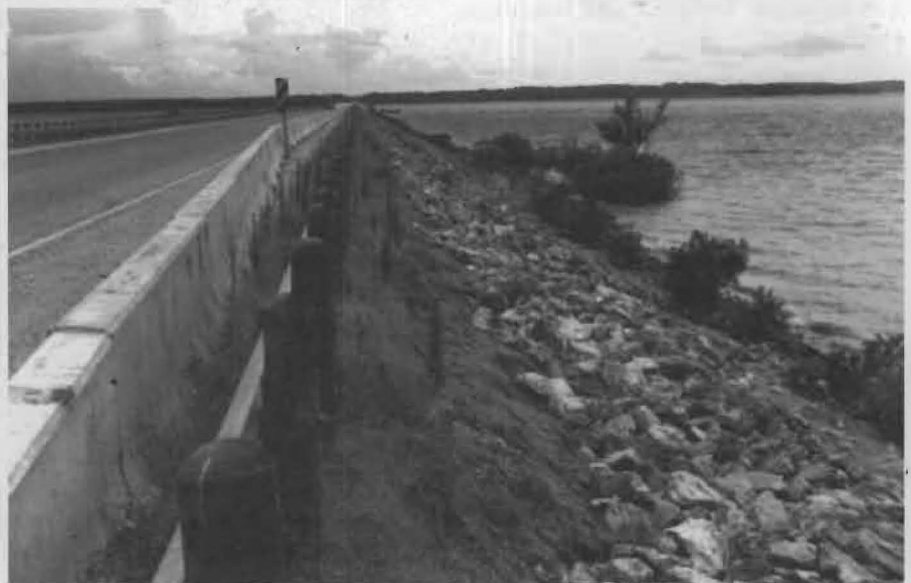
FIGURE 3: SH 147 embankment, July 1992.
