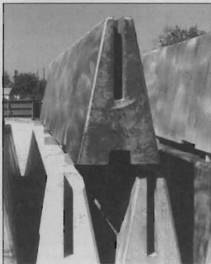
FIG. 10: Precast units in casting yard.
