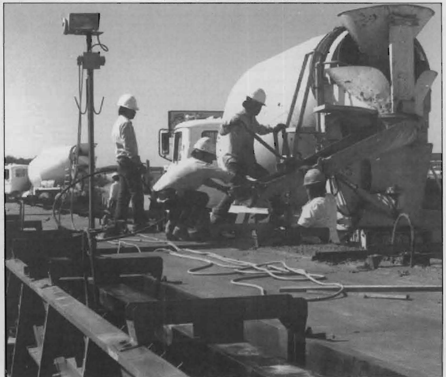
FIGURE 9: Filling the forms.
