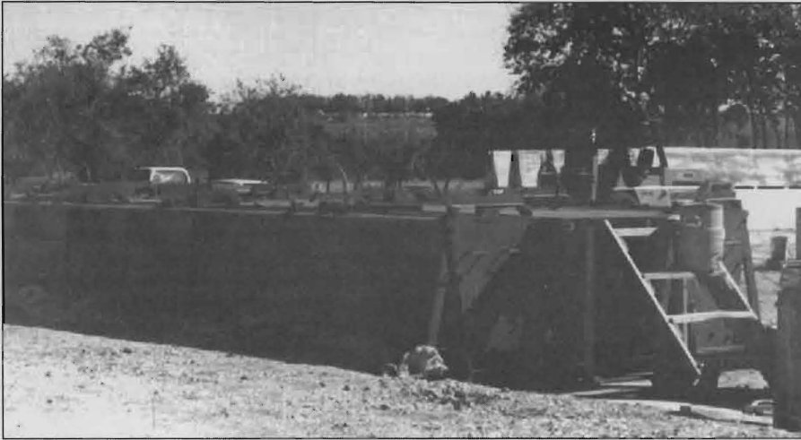
FIGURE 8: Steel form with removable end.
