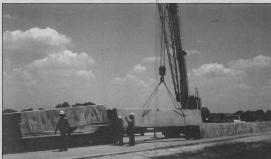
FIGURE 11: 35-ton crane placing precast barriers.
