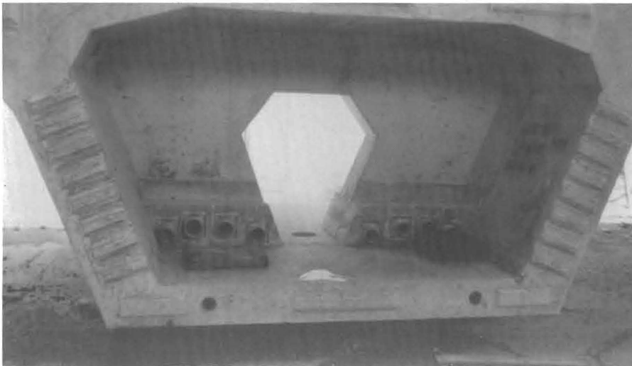
FIGURE 5: Detail of a match-cast segment.
