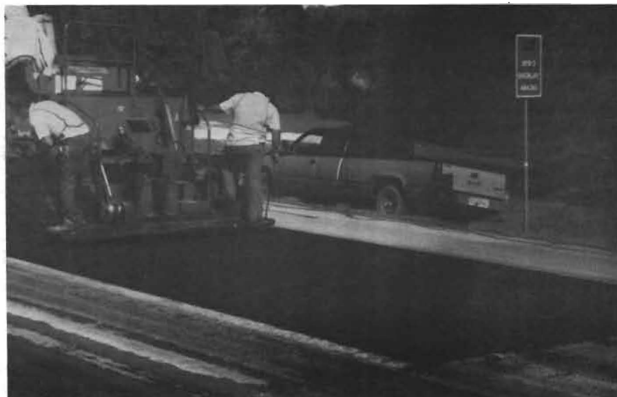
FIGURE 3: Construction of an SPS-3 site in District 15.
