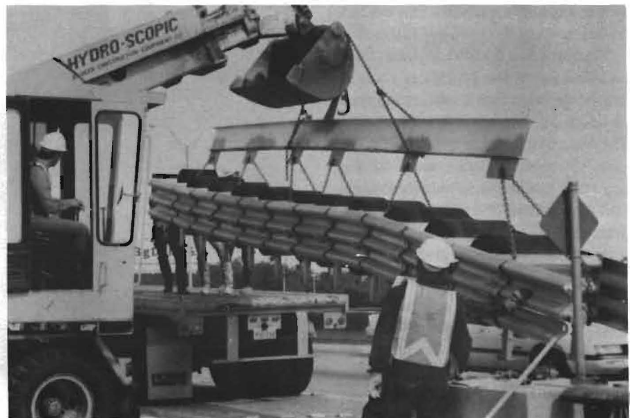
FIG. 8: Swinging the preassembled unit into place 10/31/89, IH-35.
