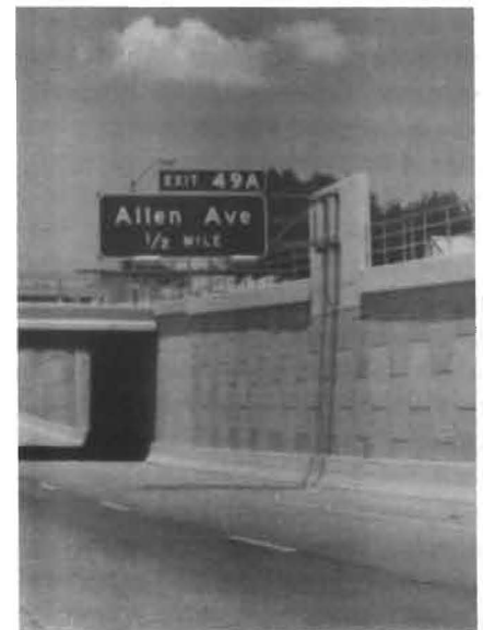
FIG. 6: Side-mounted sign on retaining wall.
