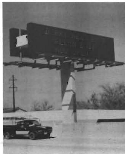
FIG. 5: Support structure for changeable message sign.
