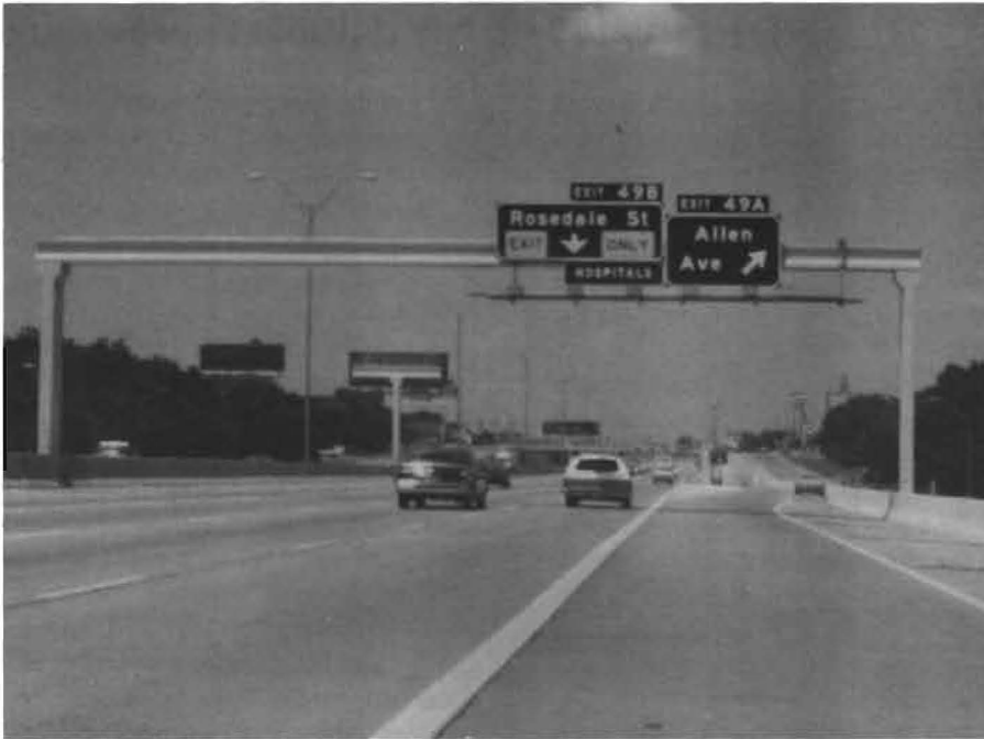
FIGURE 3: A slender concrete sign bridge.
