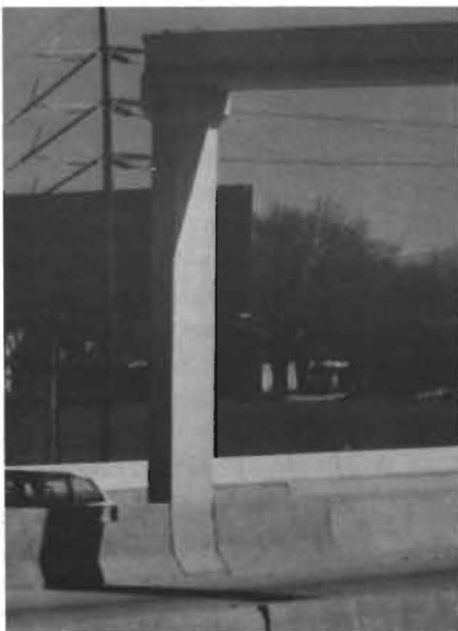
FIG. 4: Footing flush with median barrier.
