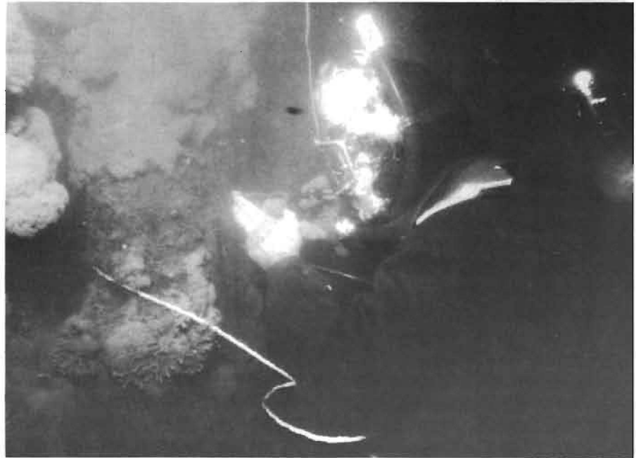
FIGURE 1: Engineer/diver inspecting underwater structure.
