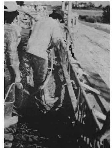
FIG.4: Using hand-held spud in congested reinforcement area.
