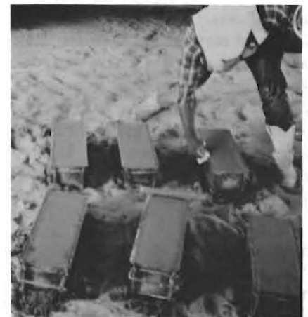
FIG.11: Casting extra beams at point of difficulty.
