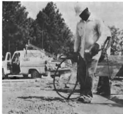
FIG.10: Vibrating along form to prevent honeycombing.
