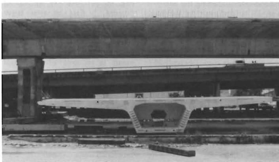
FIGURE 2: Y-wing segmental bridge in San Antonio. Most precast, prestressed elements were cast using HRWR high strength concrete.
