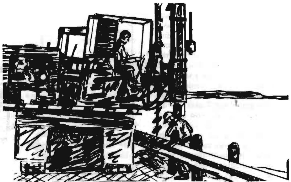
FIG.1: Truck-mounted drilling and pile-driving rig.
