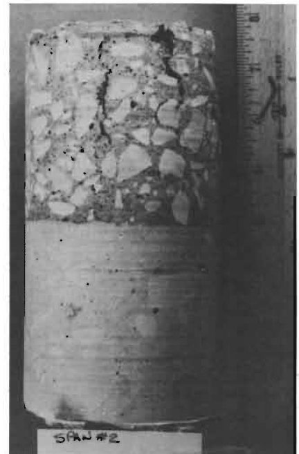
FIG. 4: Side view reveals the depth of damage.
