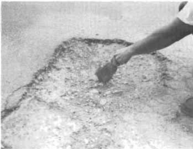
FIGURE 3: Sweep out loose debris.
