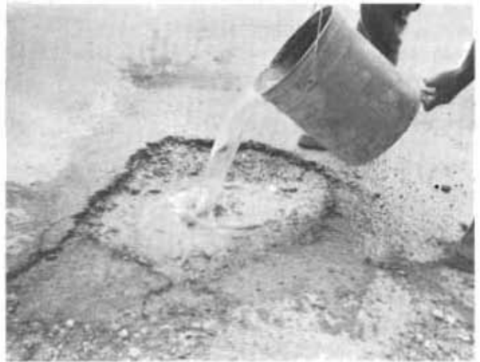
FIGURE 4: Check water level.
