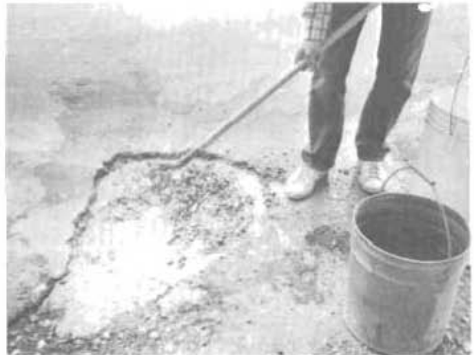
FIGURE 6: Stir while adding fly ash.
