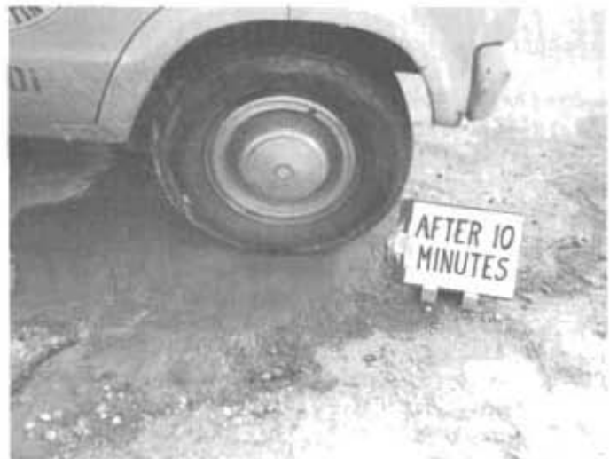
FIGURE 8: Allow fly ash to harden.
