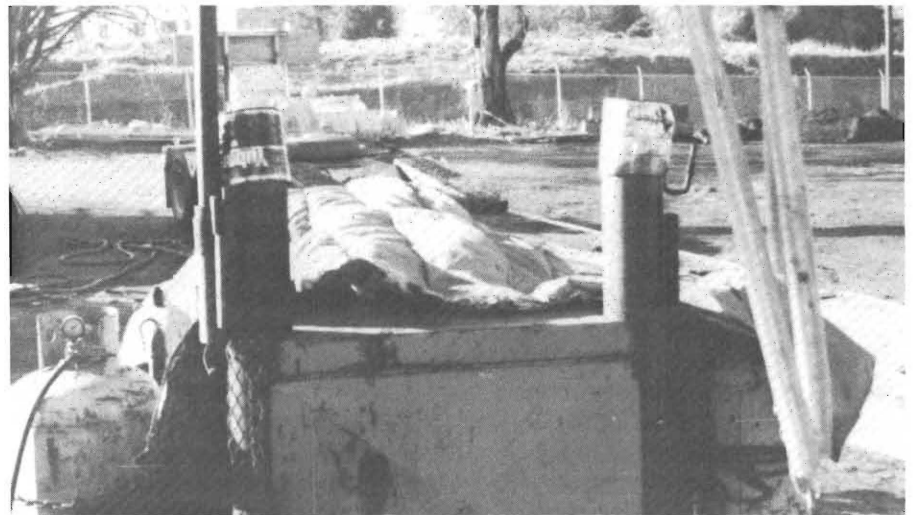
FIG. 3: Coffee cans and insulated blanket save heat.
