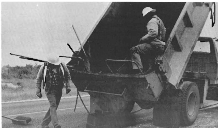
FIGURE 3 The slide or spreader box in position.
