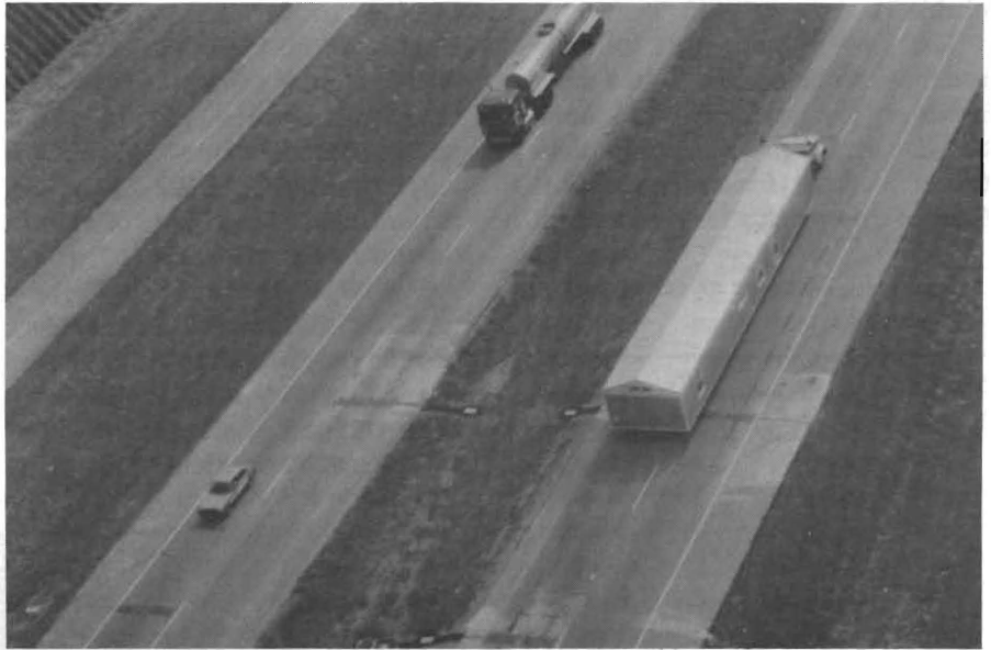
FIGURE 1 Multilane WIM installation.
