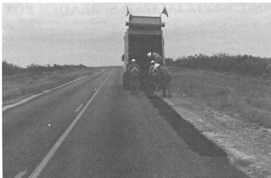
FIGURE 4 In action laying cold mix.
