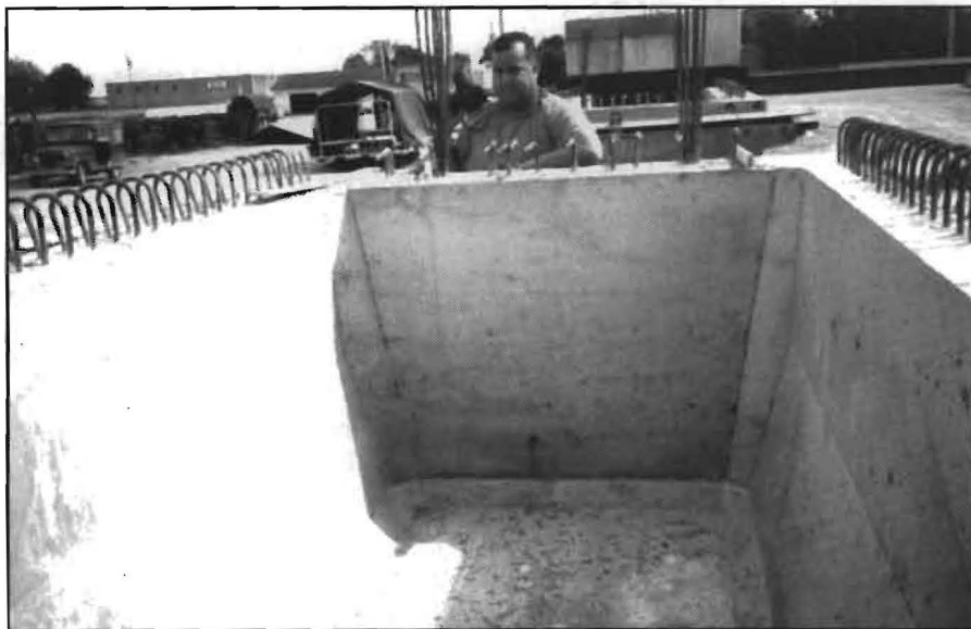
FIG. 1: Interior of U-beam at precast plant.
