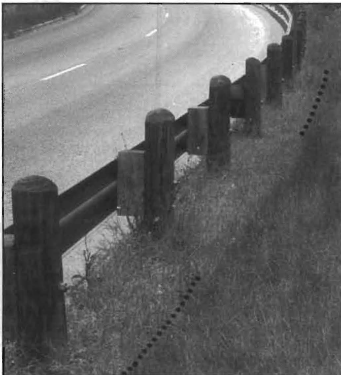
FIG. 2: Weed Blocker under 50.8 mm (2 inches) of limestone base. Dotted line indicates the approximate edge of the material.
