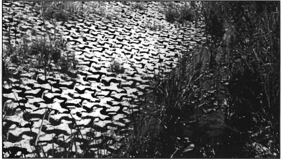
FIG. 1: The Tri-Lock erosion control system in place in Tyler District.
