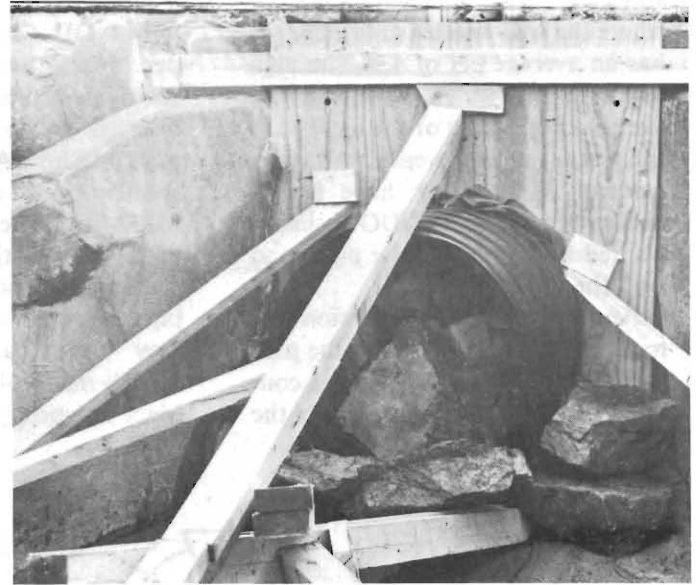
Downstream end braced and weighted.
