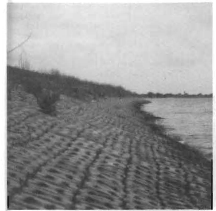
Flexible concrete riprap mat in place.
