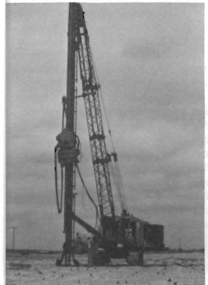
Crane with frame and mandrel for drilling wick drains.
