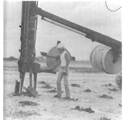
Placing wick drains.
