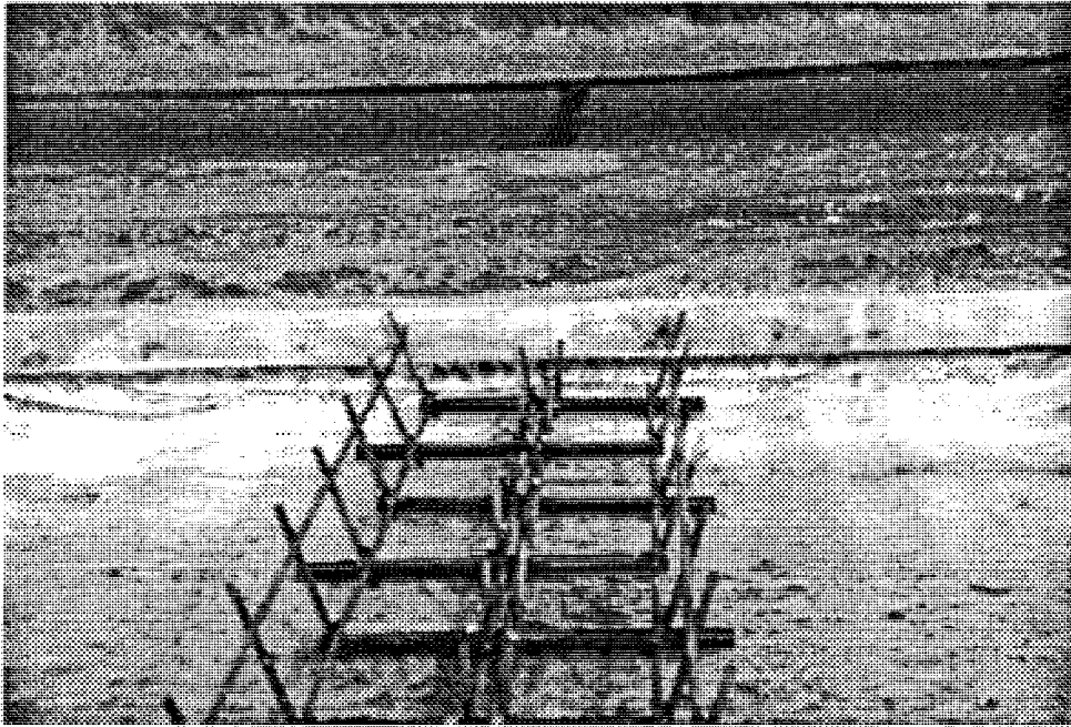
Figure 2.8 Milled joint and dowel basket assembly
