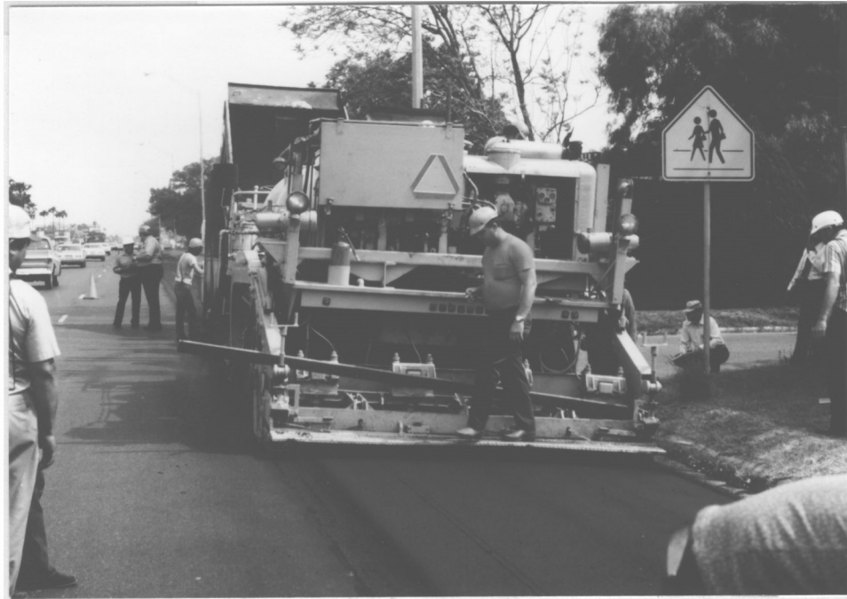
FIGURE 6 LAYING THE RECYCLED ASPHALTIC CONCRETE MAT
