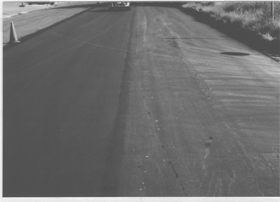
FIGURE 7 COMPLETED RECYCLED ASPHALTIC CONCRETE PAVEMENT SURFACE
