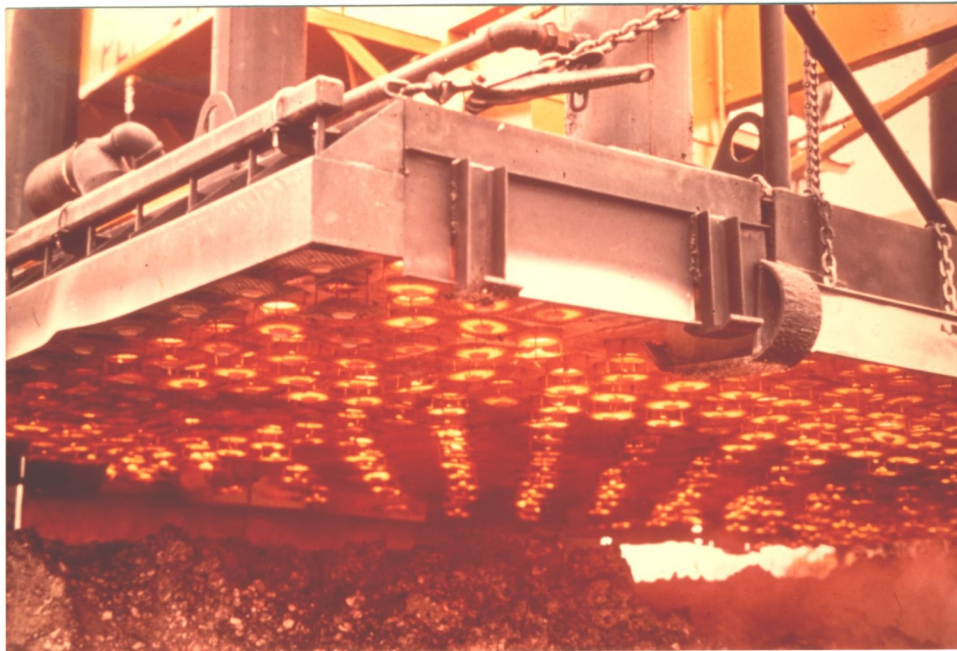
FIGURE 3 THE RADIANT HEATERS
