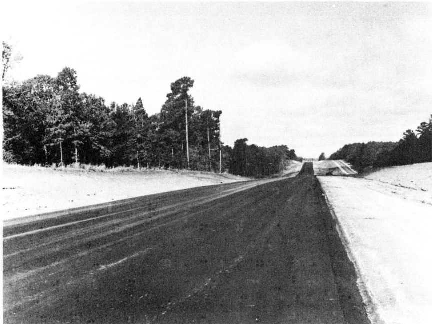
Figure 24. Completed test section prior to laying surface course.
