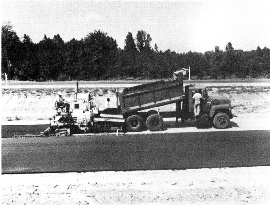
Figure 19. Placing 2-inch thick "Hot Sand" working platform over lime-stabilized subgrade.
