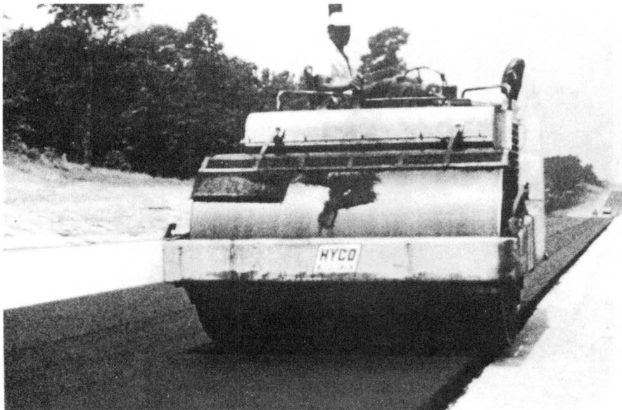
Figure 22. Hyster vibratory steel roller for initial compaction of base course.
