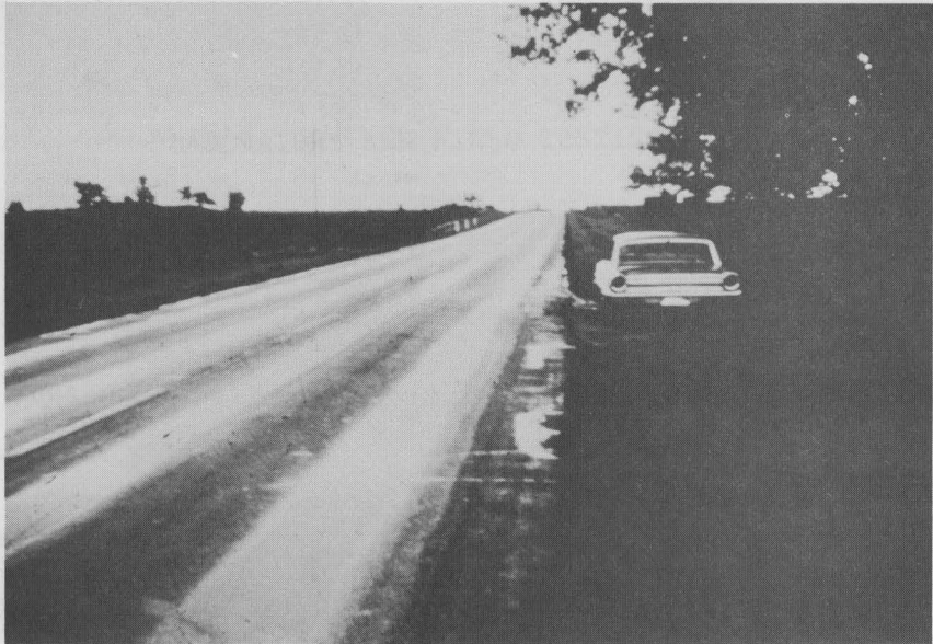
Figure 17. Wheel track depressions collect excessive amounts of water and increase the probability of dynamic hydroplaning. Such surfaces require thicker than usual overlays.
