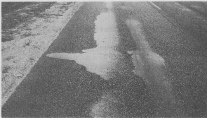
Figure 4. Flushed areas caused by fat spots in underlying pavement.
