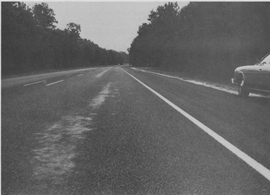
Figure 17. Wheel track depressions collect excessive amounts of water and increase the probability of dynamic hydroplaning. Such surfaces require thicker than usual overlays.
