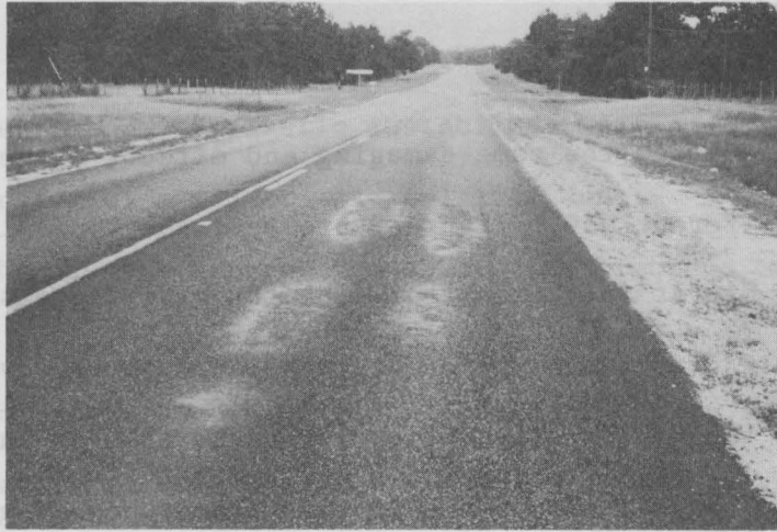
Figure 3. Evidence of delayed moisture release during construction.
