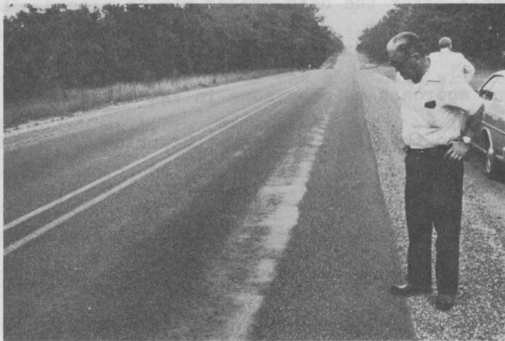
Figure 3. Evidence of delayed moisture release during construction.
