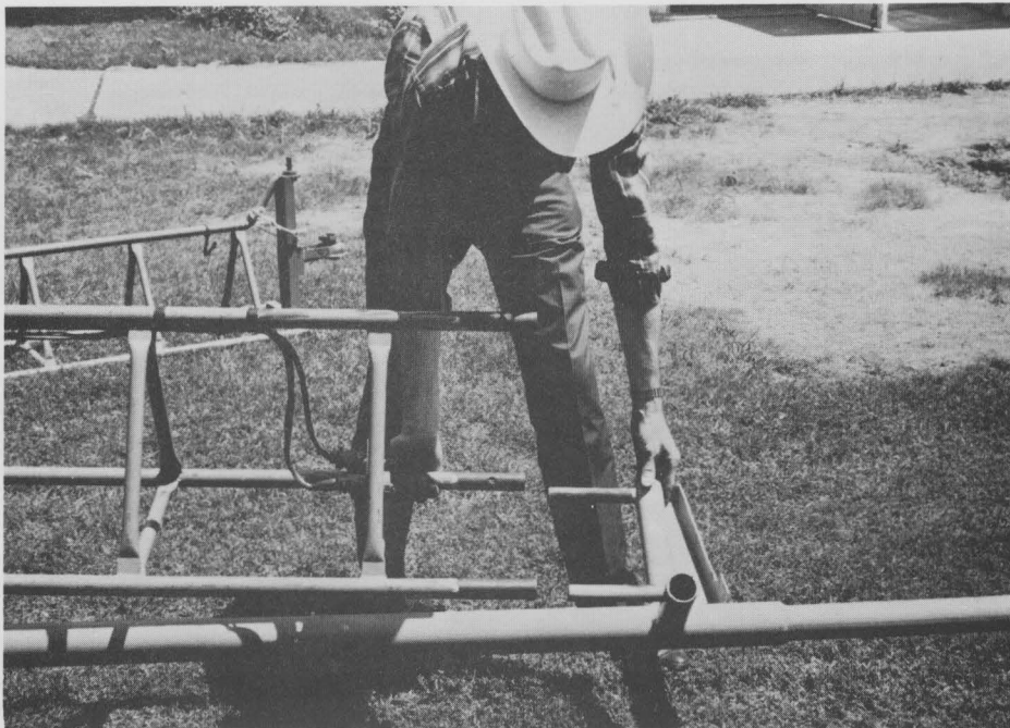
Figure 11: One-inch pipe supports being inserted into the lower legs of the rear mast section during loading operation.
