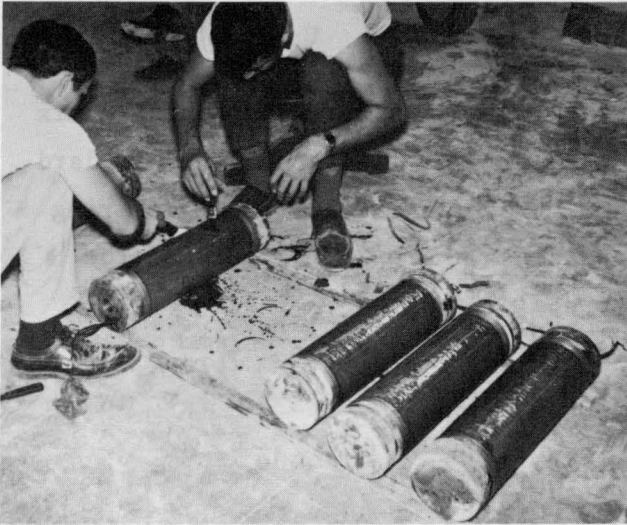
a. Application of epoxy.
