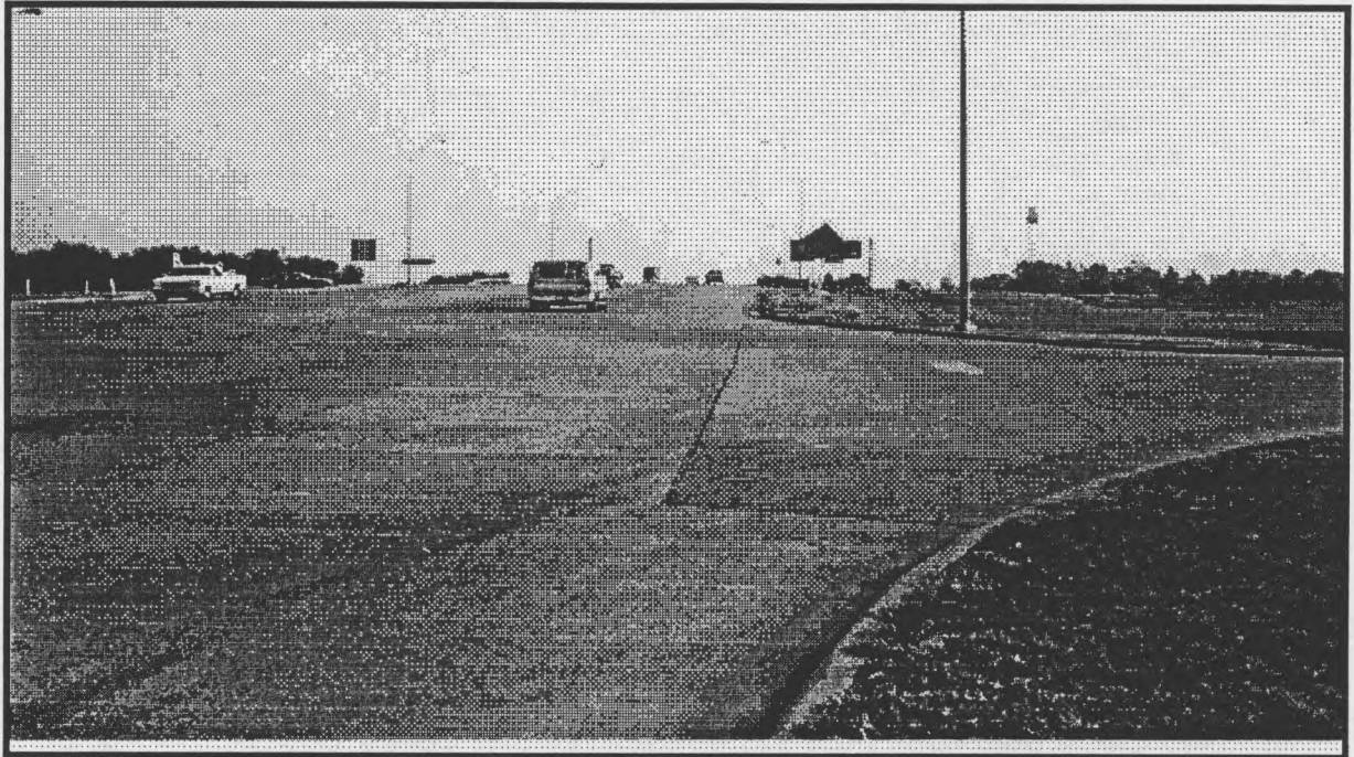
Figure 4-18a. Marshall: Looking North IH-20 / U.S. 59
