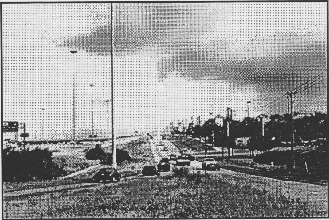
Figure 4-2a. Austin: Looking Northbound Looking North on US 183 Frontage Road Traffic Merging at Ramp and Commercial Driveways
