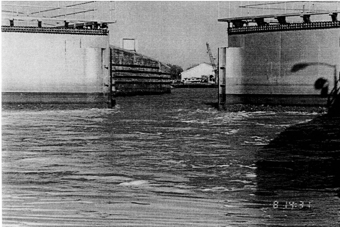
Figure E-16. Swirling current at the East Lock (east gate) while half open.
