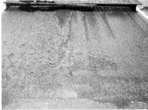
As the temperature increases, the break rate may be too fast, causing excessive drag marks and other serious problems.
