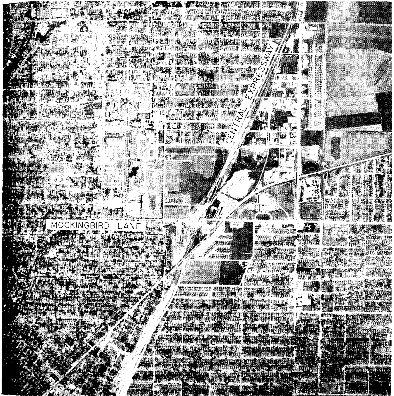
5a. Before (1951) - Central Expressway at Mockingbird Lane, Dallas
